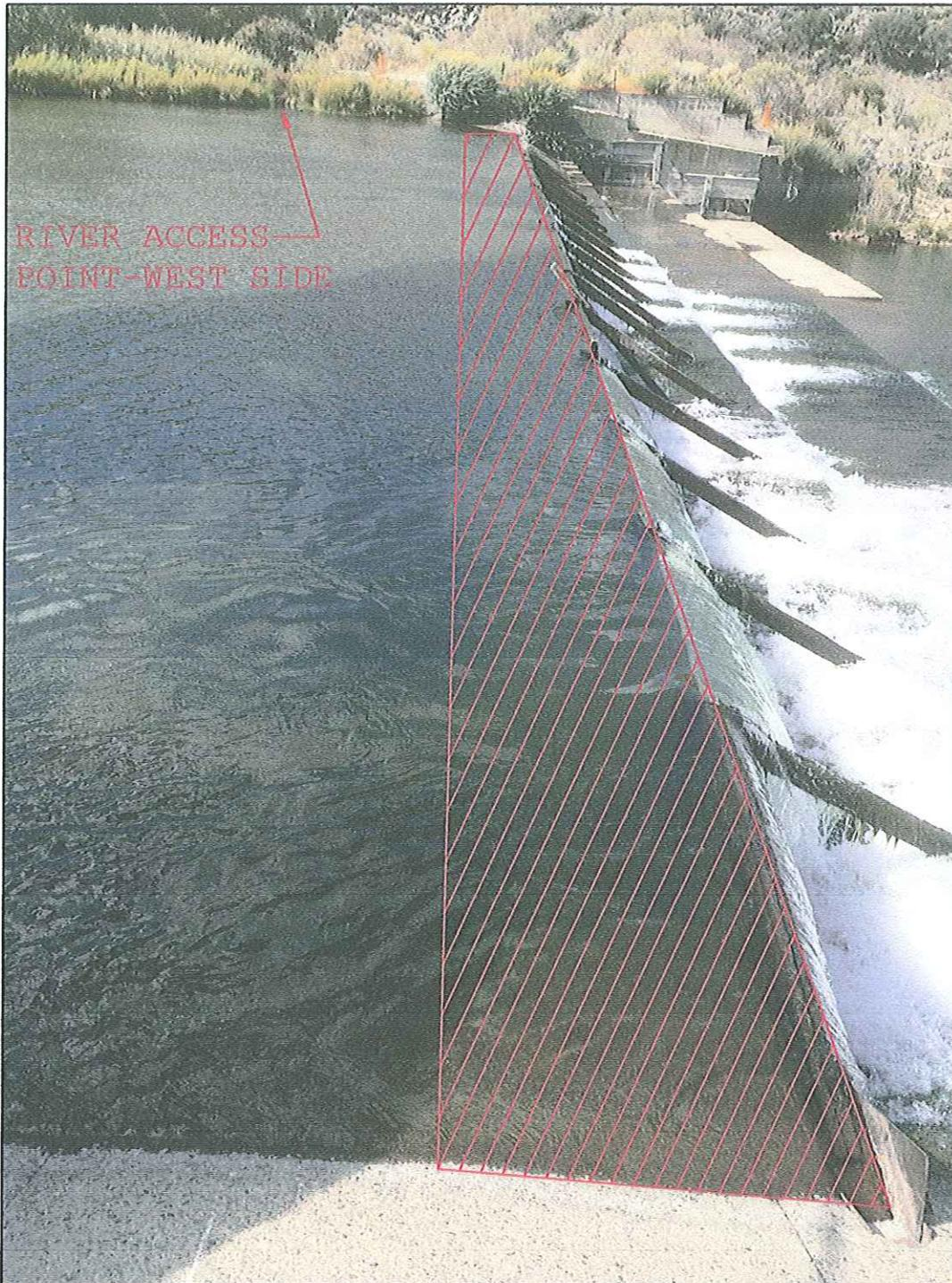
CONTRACTOR TO REMOVE AS MUCH SILT BUILD-UP FROM BEHIND THE DAM SPLASH BOARDS AS IS NECESSARY TO REMOVE AND REPLACE ALL SPLASH BOARDS AND STOP LOGS AT TOP OF FISH LADDER.
