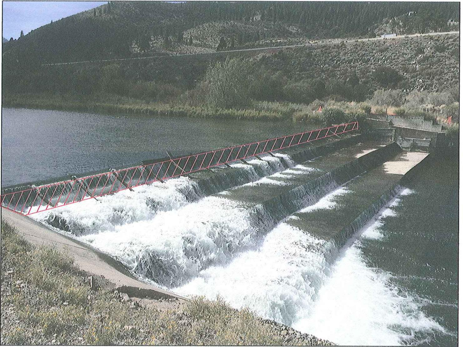
REPLACE ALL SPLASH BOARDS ON TOP OF DAM. SPLASH BOARDS ARE 3"X12"X8'. (CONTRACTOR TO VERIFY REQUIRED LENGTHS)
