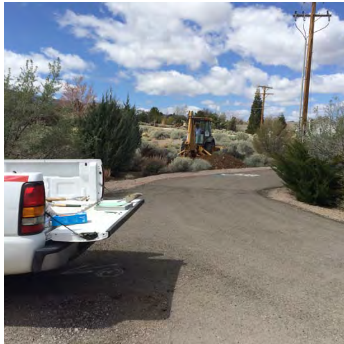
Photograph 3: Taken looking northwest toward Test Pit TP-6, located on the west side of the entrance loop.
