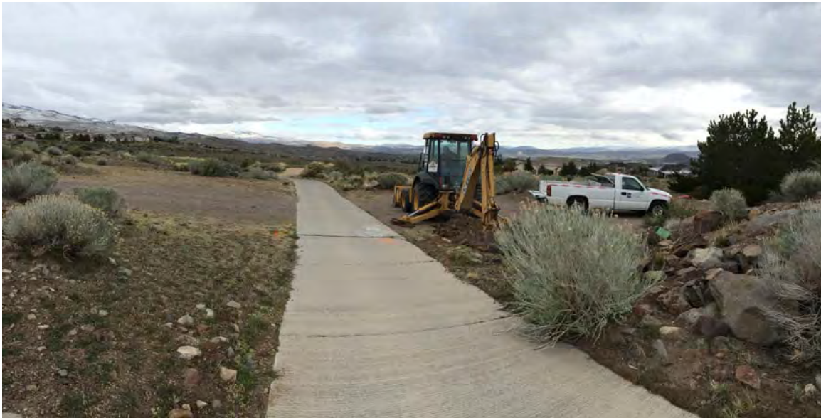
Photograph 1: Taken looking north toward Test Pit TP-1, note embankment masking existing well house facility.
