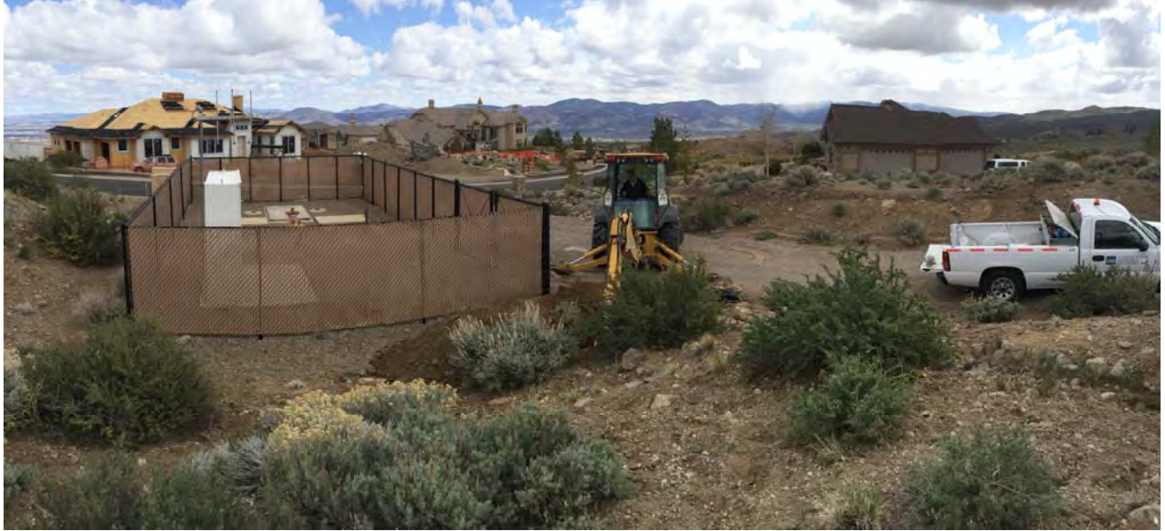
Photograph 2: Taken looking north toward test pit TP-4
