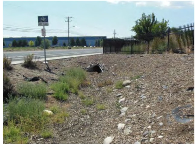
Photo #2: Looking south along existing drainage ditch.
