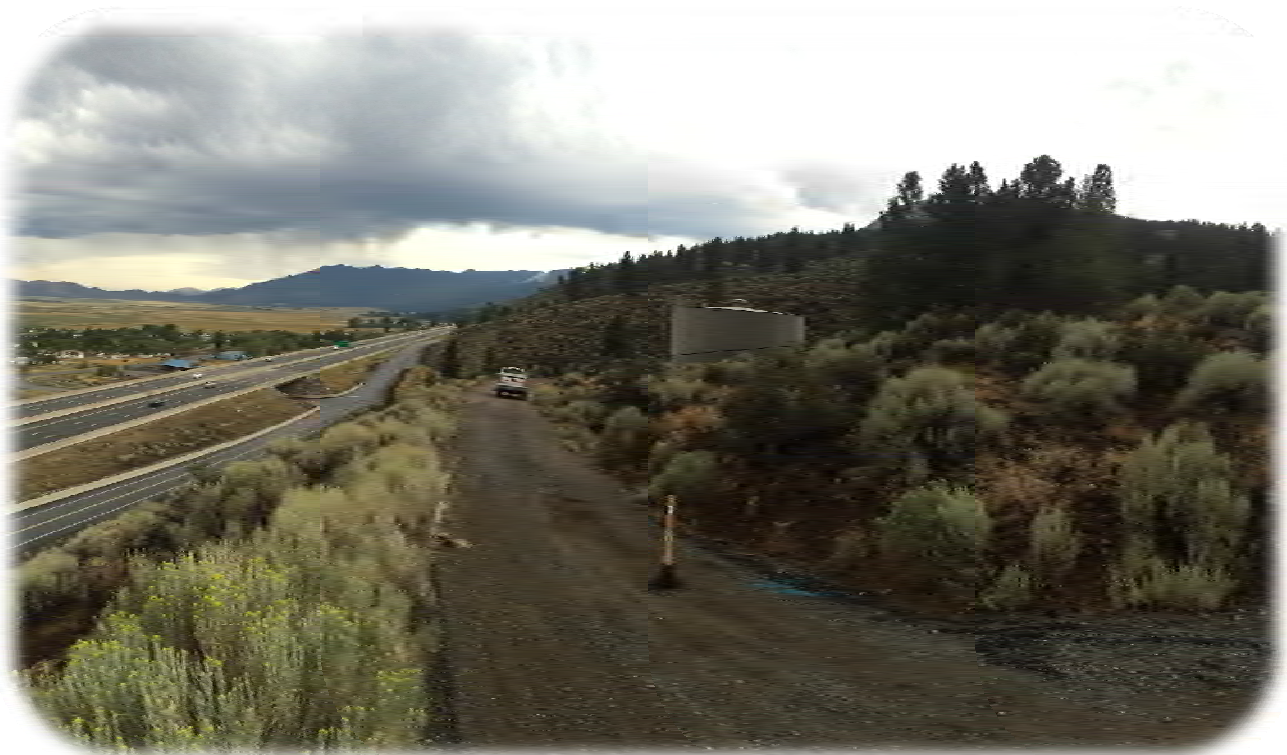
Photograph 1: Taken looking south toward Test Pit TP-2. Test Pit TP-1 is located south of TP-2 near the pictured service vehicle.
