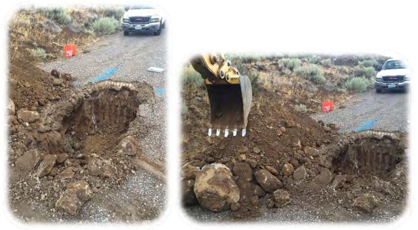
Photographs 2 and 3: Taken looking northwesterly toward Test Pit TP-1. Note large cobbles and boulders encountered below a depth of 1 foot to the depth of exploration.
