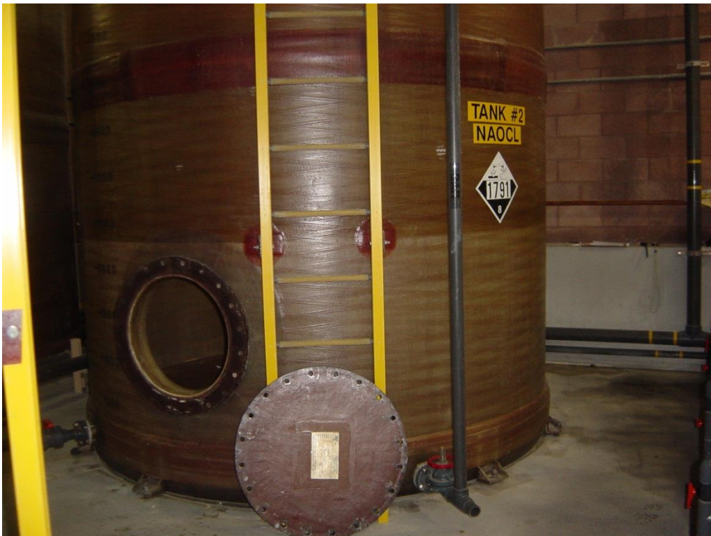
Exterior representation of Chalk Bluff Tanks #3 & #4 depicting 24" man-way and ladder
