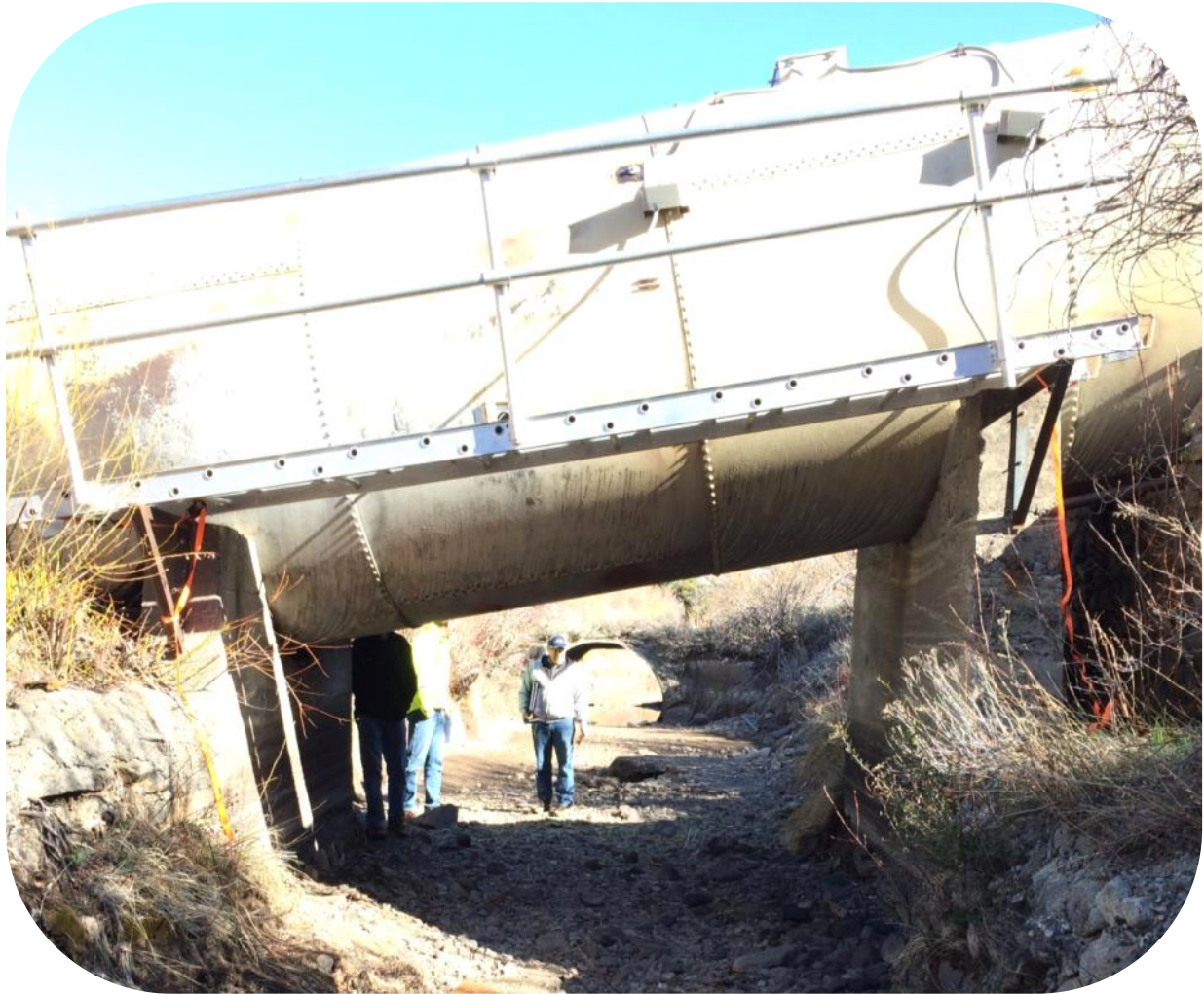
Photo #2: Looking north at existing penstock from bottom of Steamboat Ditch
