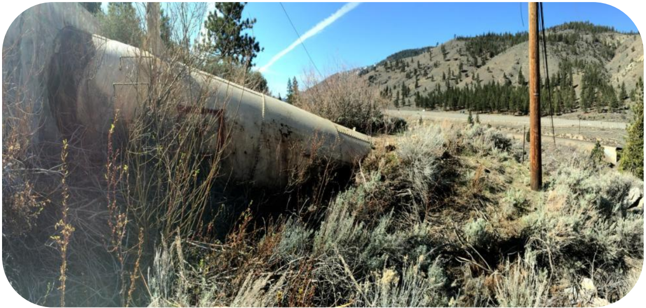
Photo #4: Looking south showing fill embankment near penstock connection to the Forebay
