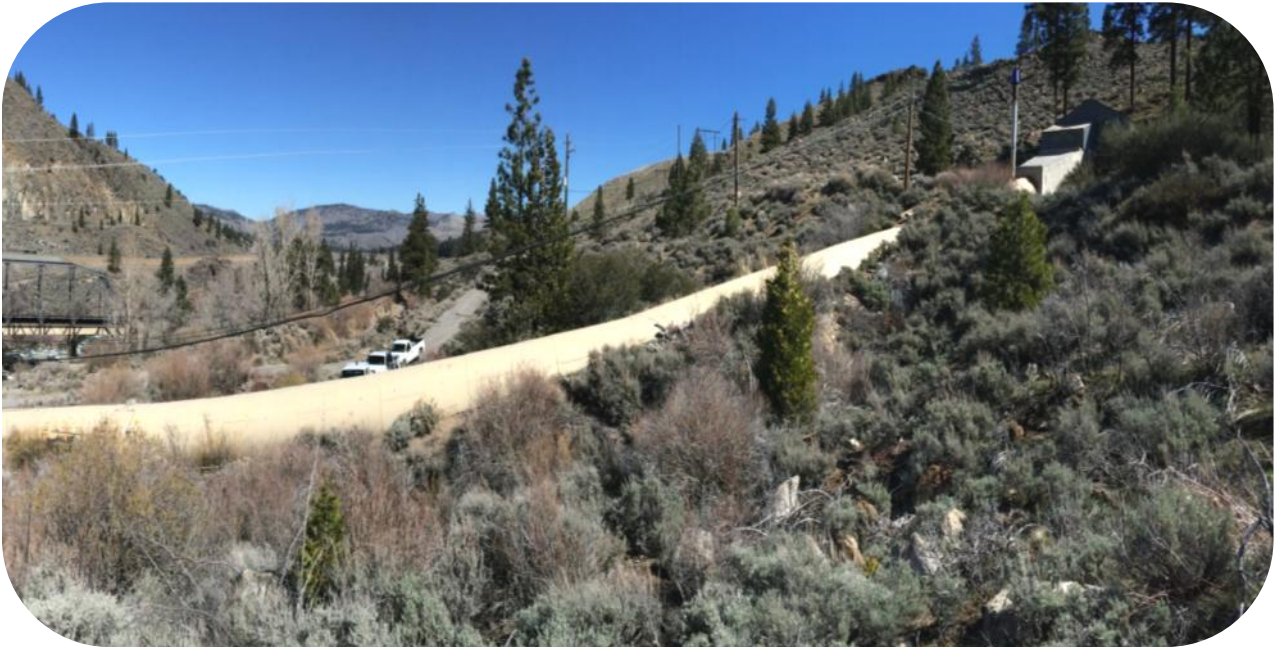
Photo #5: Looking north showing existing terrain adjacent to the existing penstock east of Steamboat Ditch
