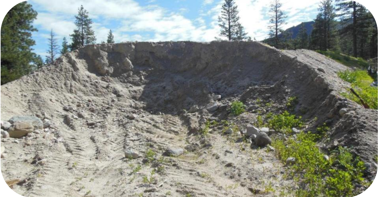
Photo #6: Looking east at west end of soil stockpile
