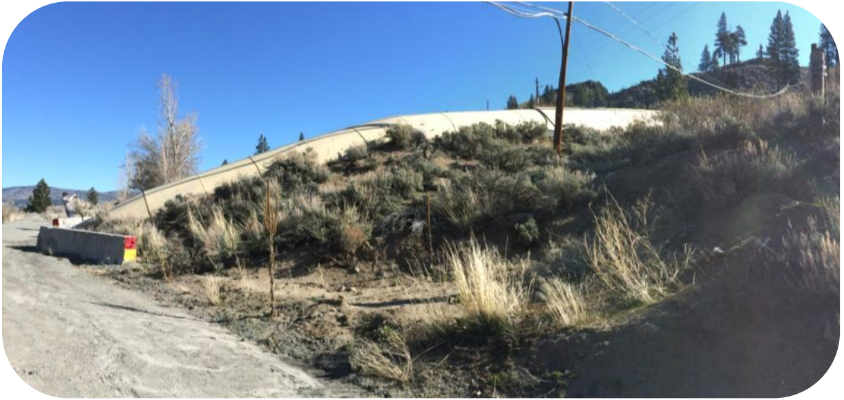
Photo #3: Looking north showing existing penstock descending below the access road
