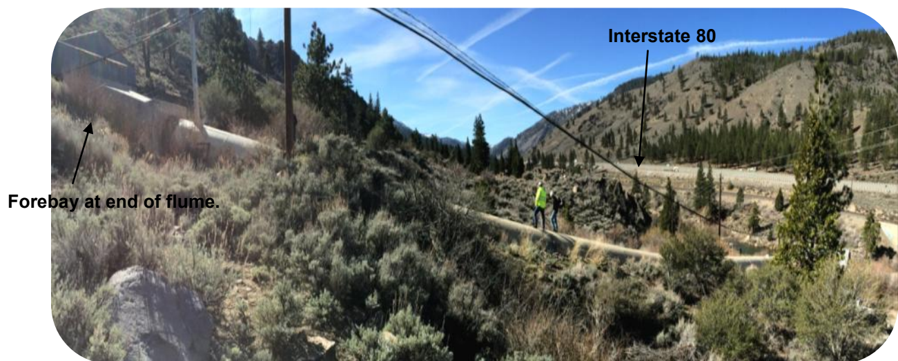
Photo #1: Looking south at existing penstock from access road.
