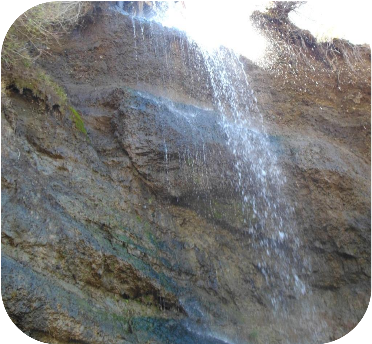
Photo #2: Showing uppermost exposed volcanic bedrock directly below end of existing spillway channel
