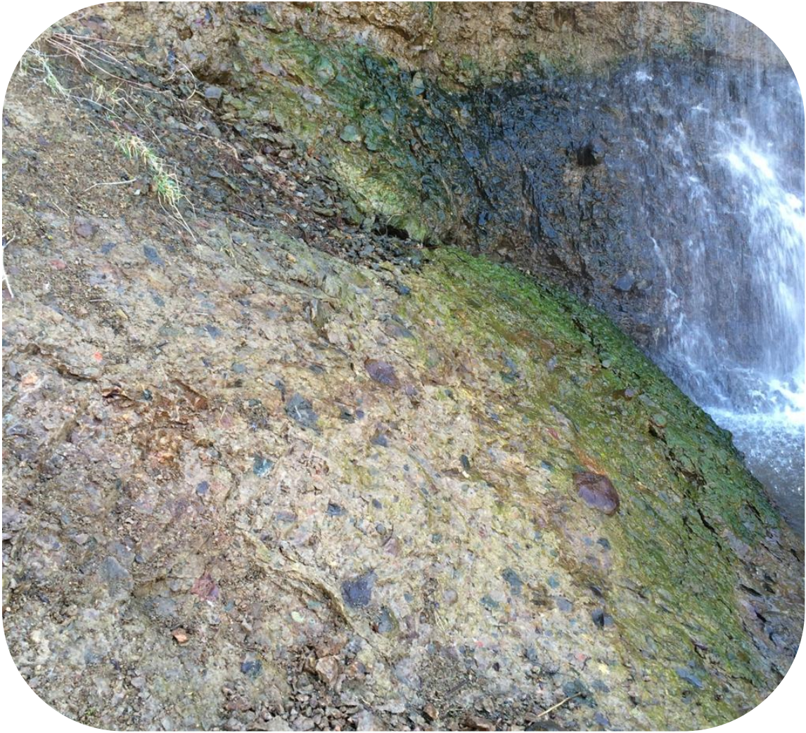
Photo #3: Showing lowermost exposed basaltic bedrock directly below end of existing spillway channel. Note angular rock fragments in the bedrock indicative of a Lahar deposit.
