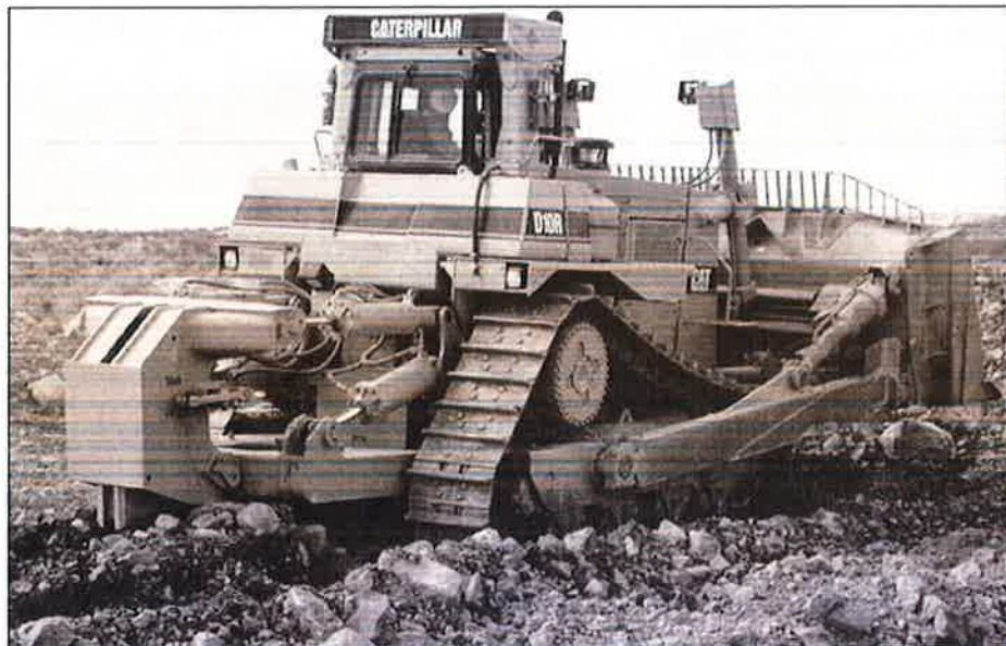
Correct dozer position during ripping process.
