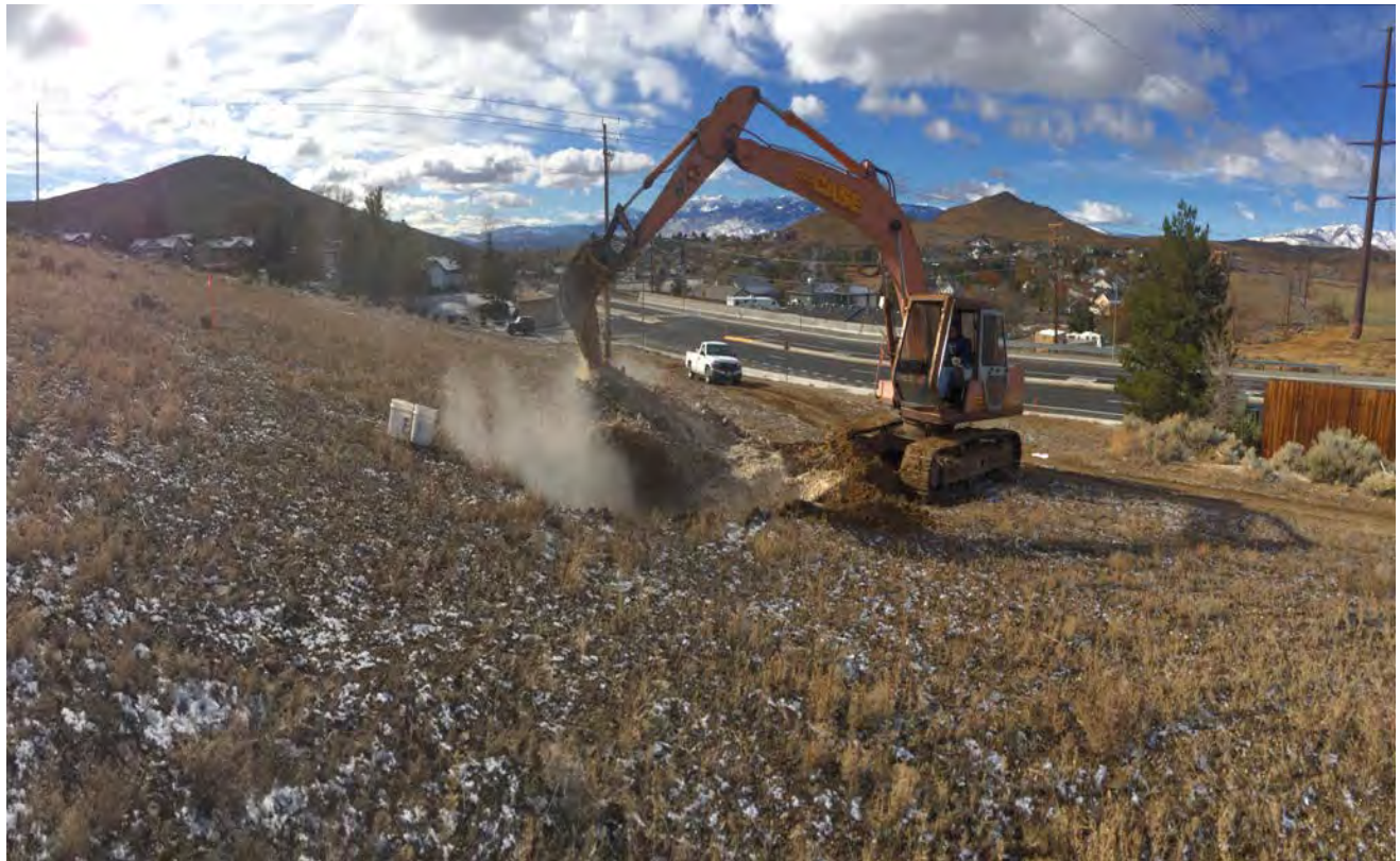
Photo #1: Looking southwest from east side of property. Note existing generator enclosure to the west.
