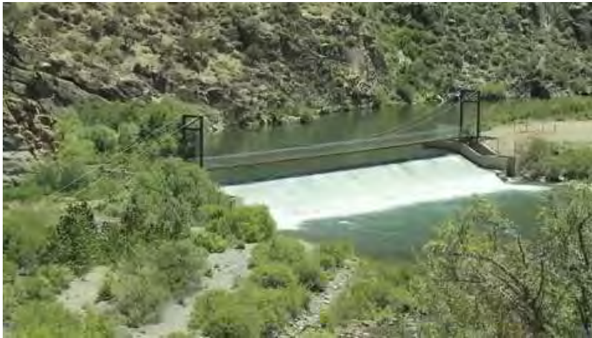
Tahoe-Pyramid Bikeway opens new bridge: Tahoe-Pyramid Bikeway opens new bridge
