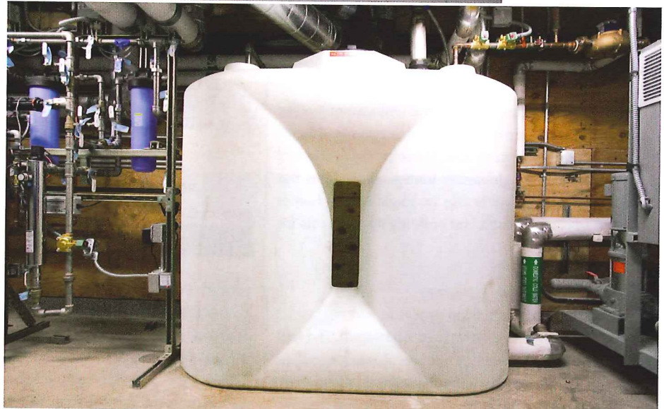
Rainwater from the Bullitt Center's roof is captured, filtered, and carried to a 56,000 gallon cistern in the basement to supply all non-potable fixtures in the building. Composting units (left) and a storage tank for rainwater that has been purified for potable use (below) are key elements in the building's treatment of wastewater.
