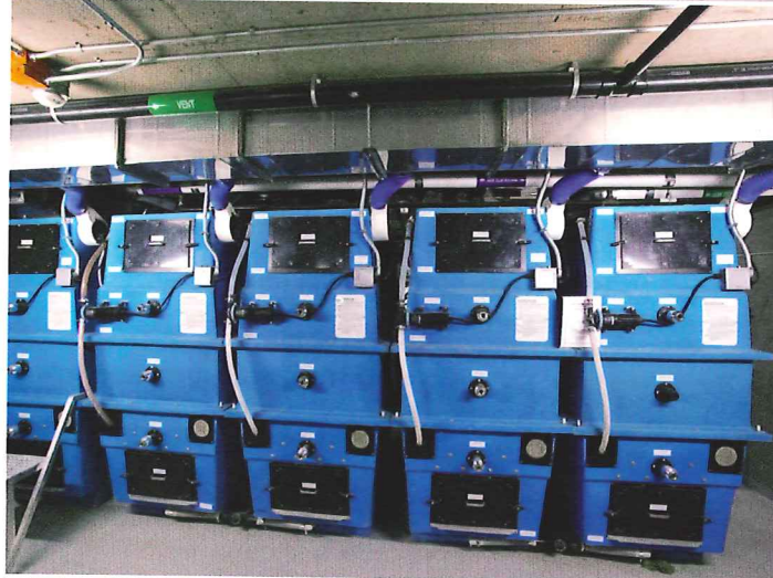
Rainwater from the Bullitt Center's roof is captured, filtered, and carried to a 56,000 gallon cistern in the basement to supply all non-potable fixtures in the building. Composting units (left) and a storage tank for rainwater that has been purified for potable use (below) are key elements in the building's treatment of wastewater.
