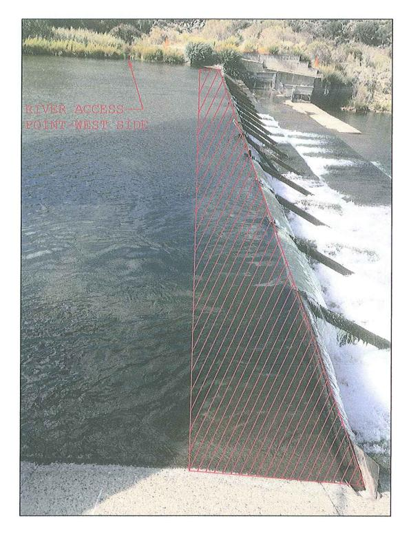
CONTRACTOR TO REMOVE AS MUCH SILT BUILD-UP FROM BEHIND THE DAM SPLASH BOARDS AS IS NECESSARY TO REMOVE AND REPLACE ALL SPLASH BOARDS AND STOP LOGS AT TOP OF FISH LADDER.
