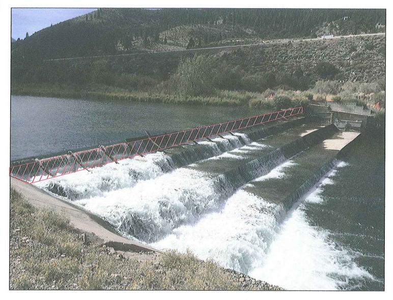
REPLACE ALL SPLASH BOARDS ON TOP OF DAM. SPLASH BOARDS ARE 3"X12"X8'. (CONTRACTOR TO VERIFY REQUIRED LENGTHS)
