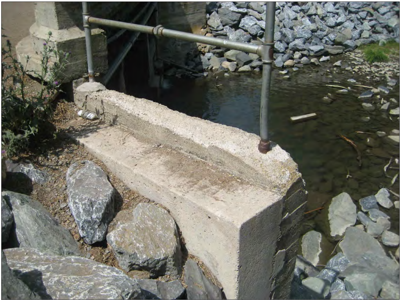
2 S4 SPALLING ON TOP OF SE WINGWALL MARK ①
