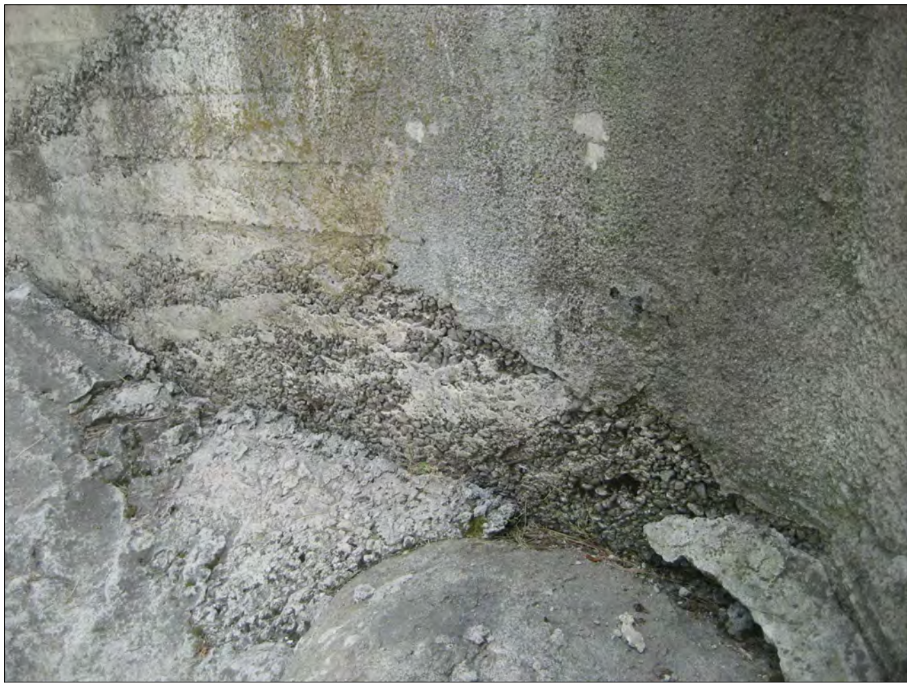
4 S4 ROCK POCKET IN FACE OF SE WINGWALL MARK ②
