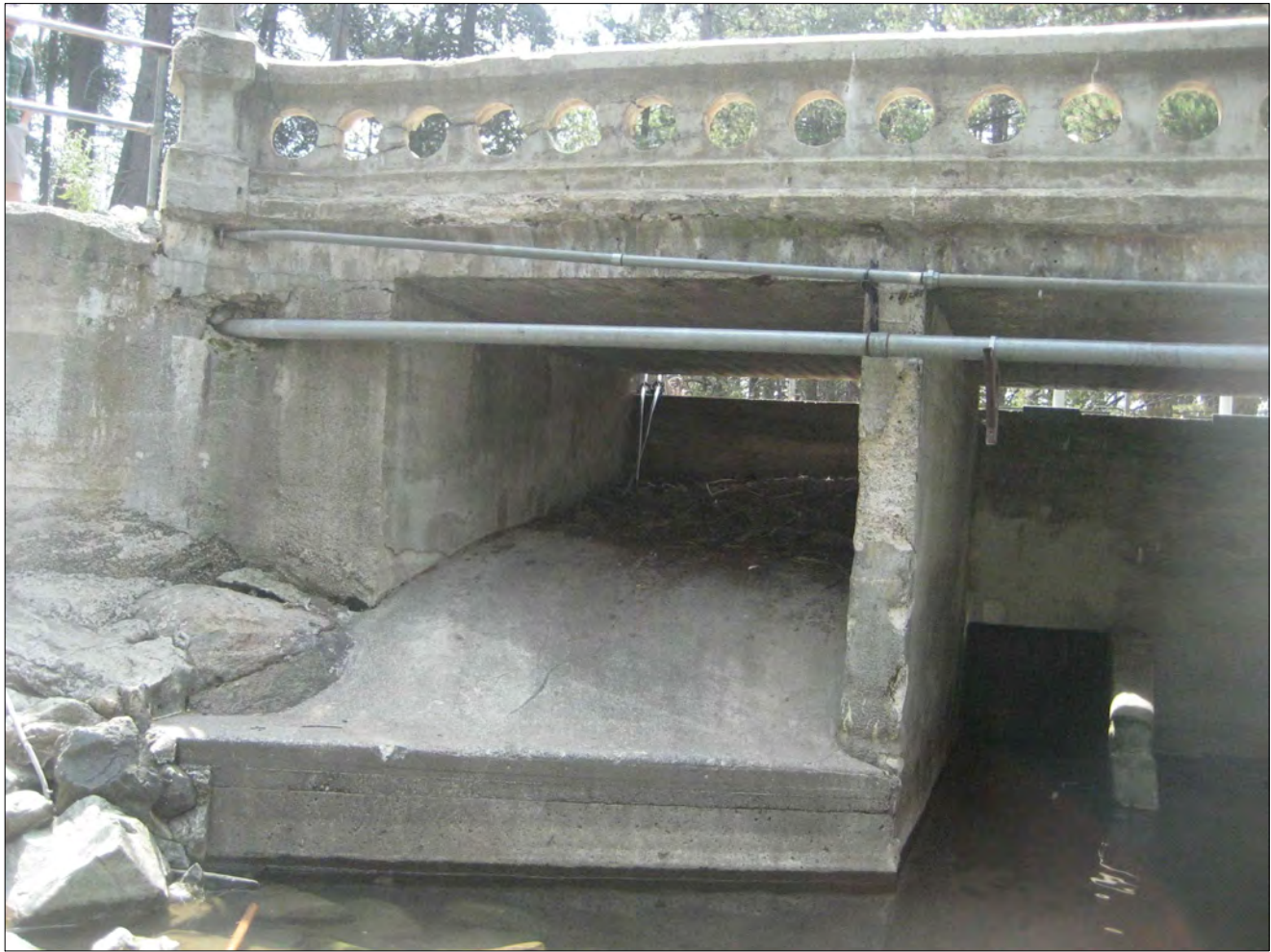
1 S4 SPALLING AT DOWNSTREAM WALL MARK ①
