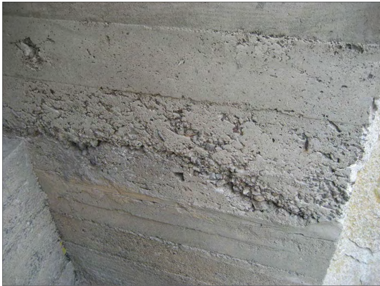
3 S4 ROCK POCKET IN NORTH WALL MARK ②
