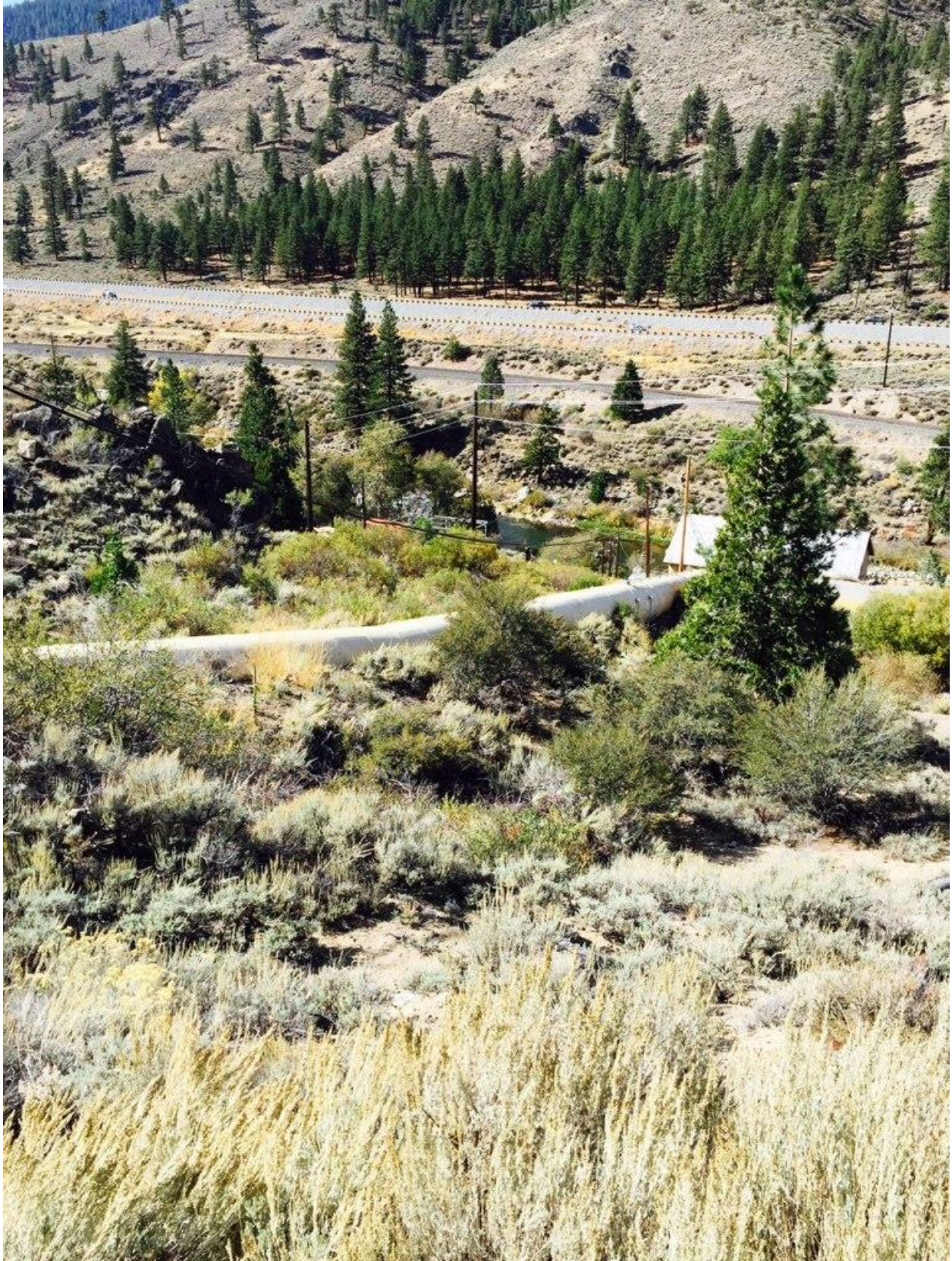
Fleish Penstock down to Powerhouse
