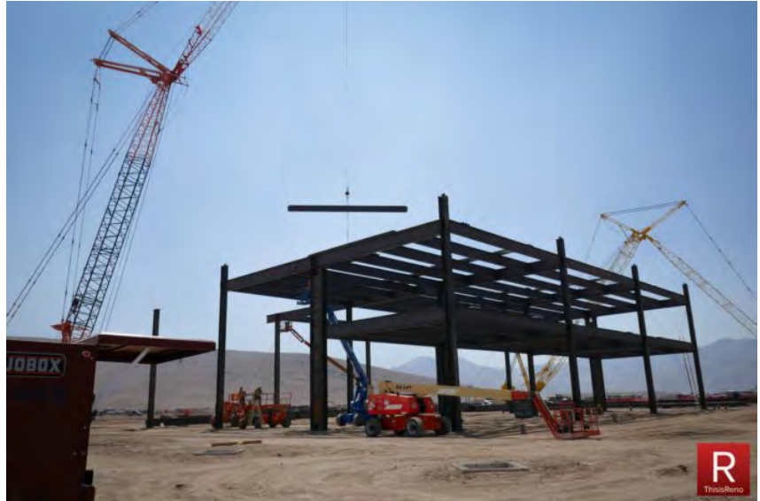
The Tesla Gigafactory under construction. Image: Bob Conrad.
