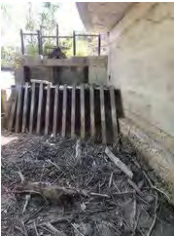
Sediment clogs Cochrane Ditch on the south side of the Truckee River near Sierra Street in downtown Reno. (Photo: Provided by Lauren Ball/City of Reno)
