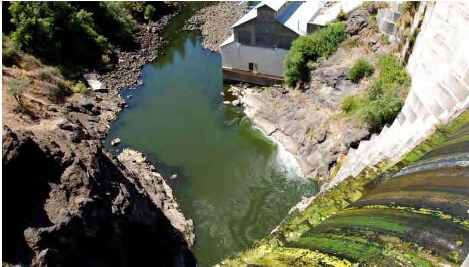
Water trickles over Copco 1 Dam on the Klamath River outside Hornbrook, Calif. on Aug. 21, 2009. (Jeff Barnard / Associated Press)
