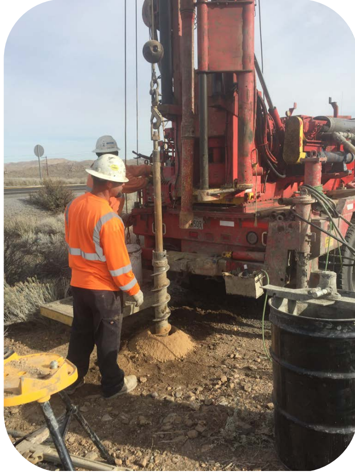
Photograph 2: Boring B-2 at a depth of about 7 ½ feet. Note cobbles present on the ground surface.
