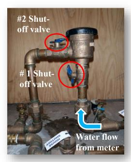
off valve should be done slowly to allow the water to gradually fill into the irrigation system. Going too quickly could be damaging to parts of your backflow.
