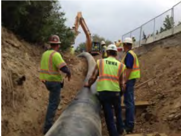
TMWA Workers Install a Water Main Pipeline. Photo:
