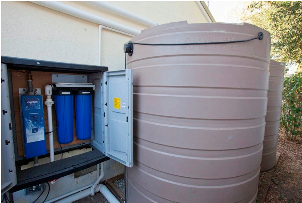
An 865-gallon rain barrel next to a water filter and micron filters for harvested rainwater on a green home in Los Angeles. (Citizen of the Planet/Education Images/UIIG via Getty Images)
