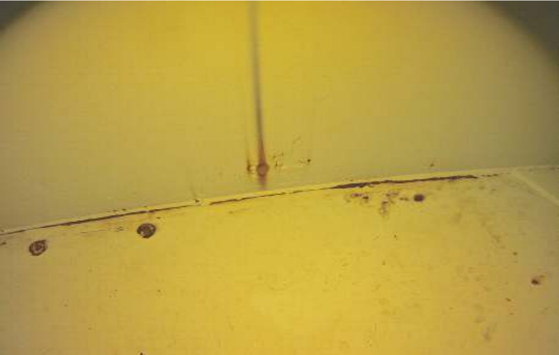
13. Floor at Shell
