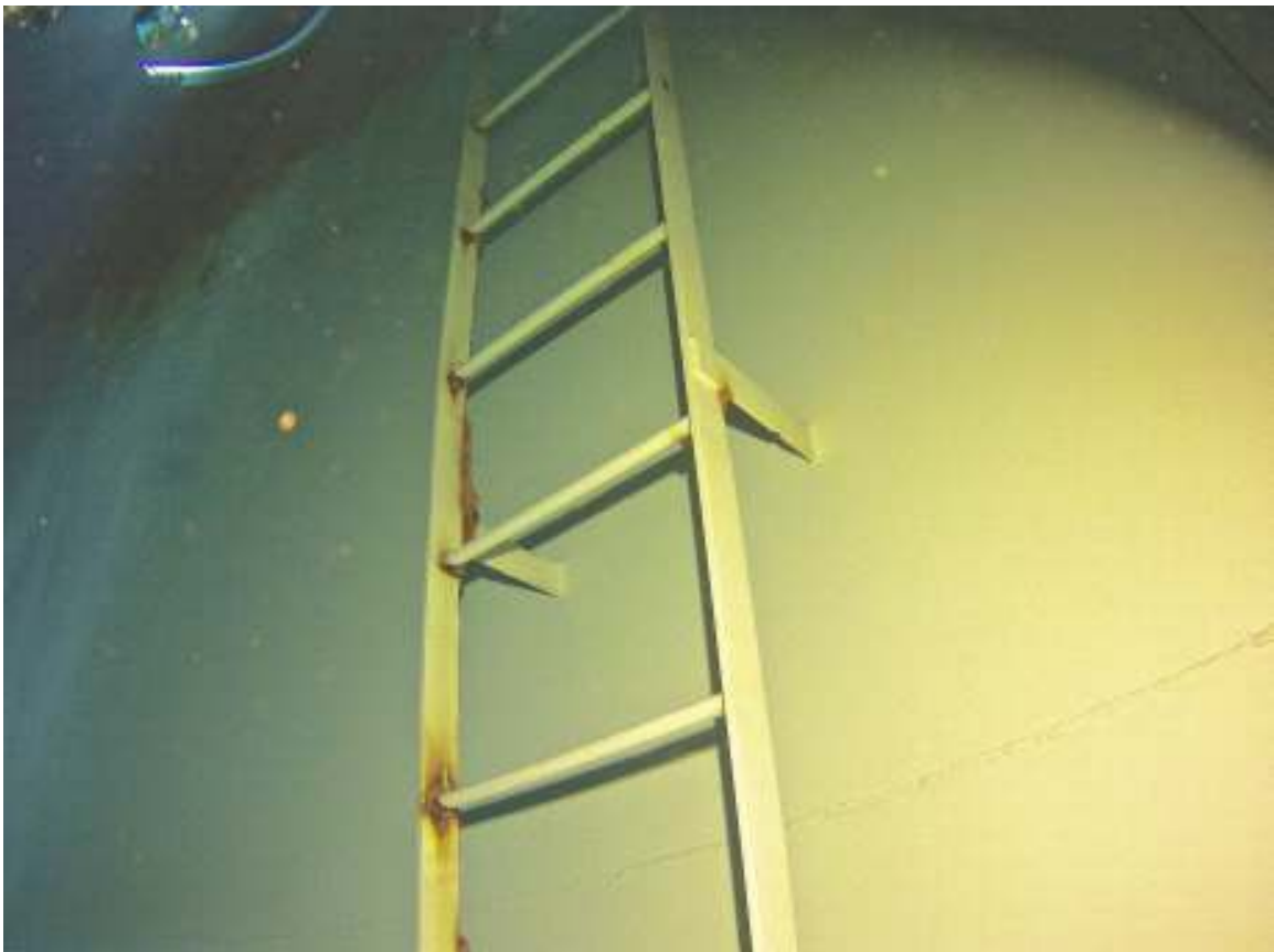
40. Interior Ladder - Middle
