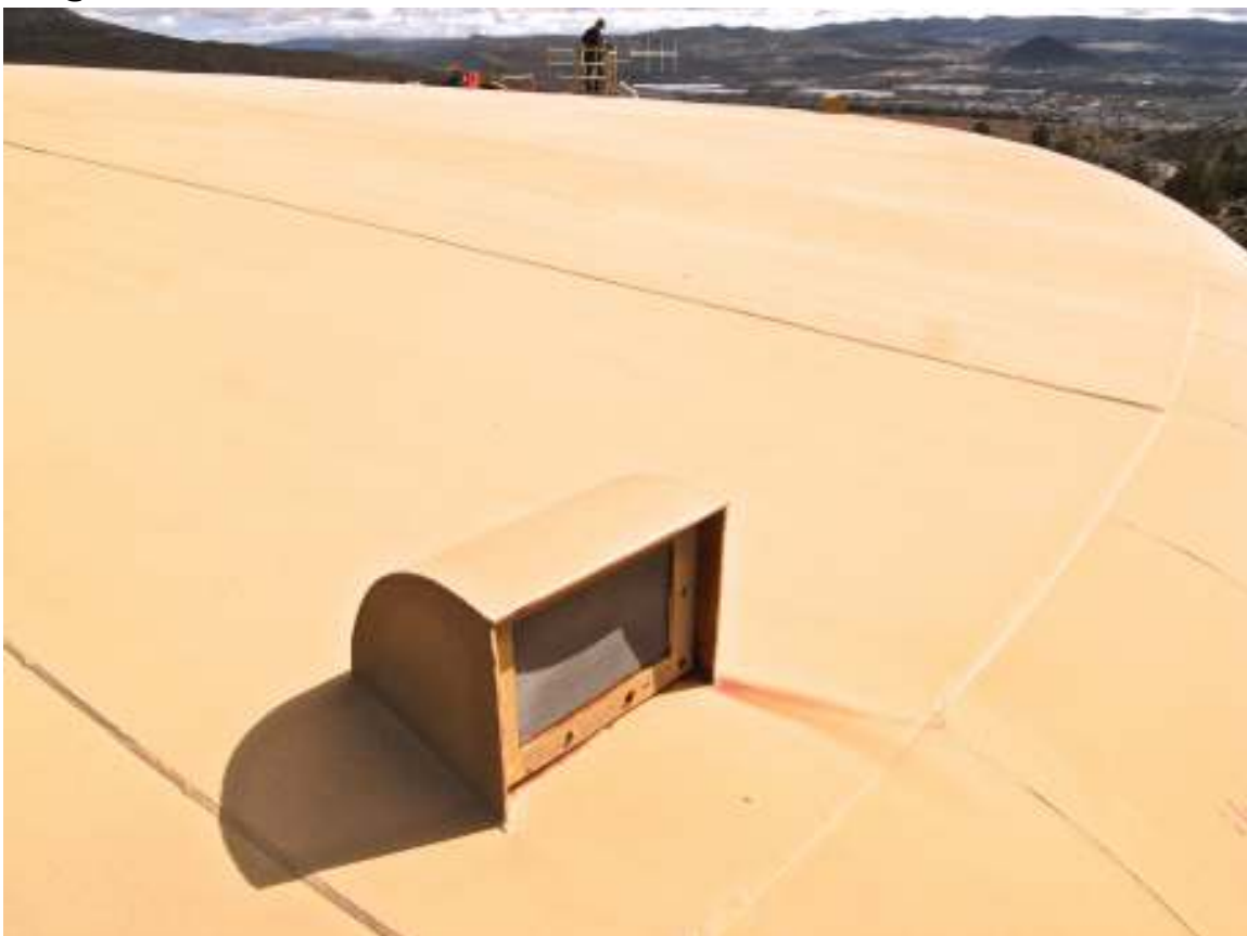
38. @1 of 6 - Perimeter Roof Vents
