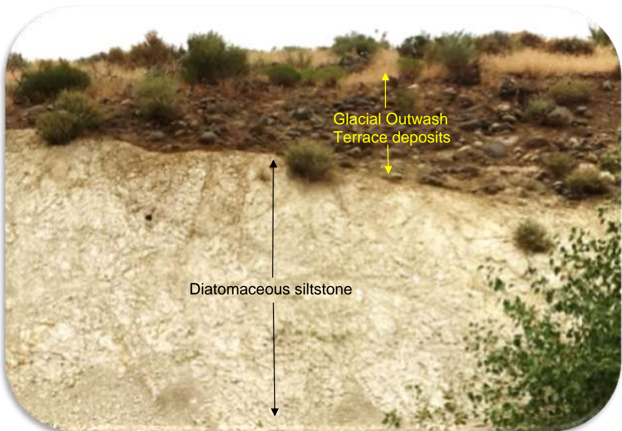
Photograph 1: Cut slope behind Highland Ditch Canal showing the different geologic units
