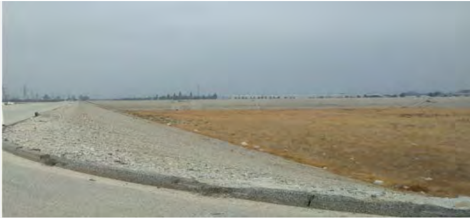
The severed pipeline at the Hansen Spreading Grounds is a reminder of and the importance of outreach.
