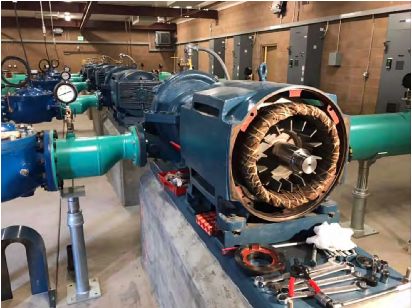
Photo Of: Pyramid - Point View Booster Pump Station Electronic Motor Bearing Replacement
