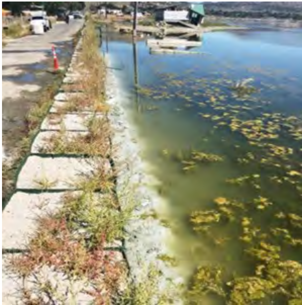
A HESCO barrier after bentonite was applied to it.
