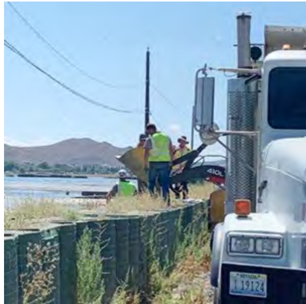
Crews apply bentonite clay to a portion of the HESCO barriers around Swan Lake on Sept. 3. COURTESY/WASHOE COUNTY
