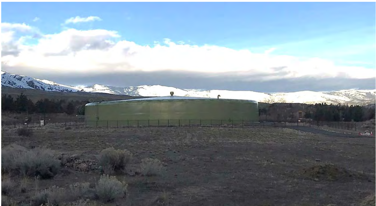
Hunter Creek Tank
