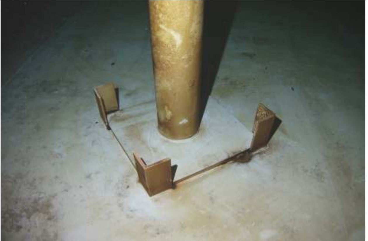
31. Perimeter Support Pole Base
