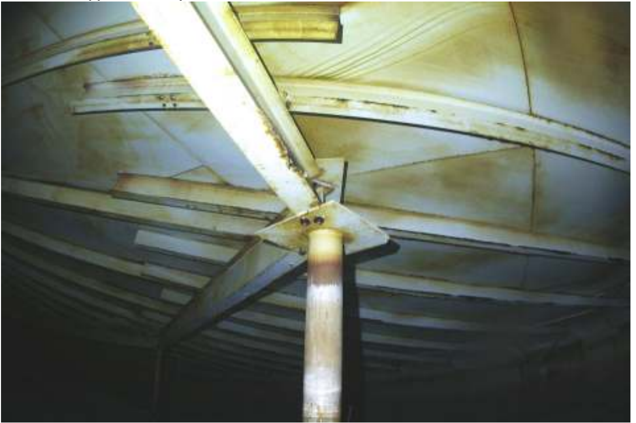
33. Perimeter Support Pole Top
