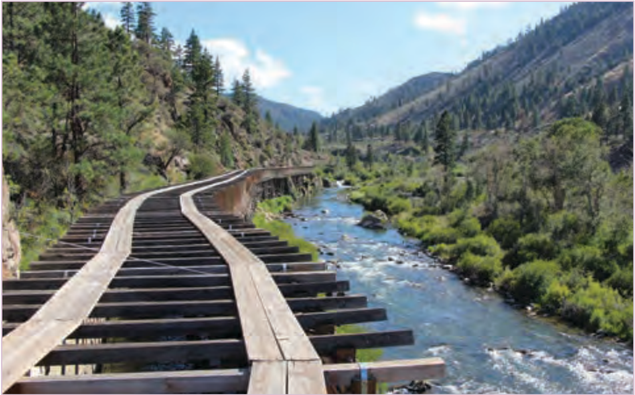
HYDROELECTRIC FLUME ALONG THE TRUCKEE RIVER
