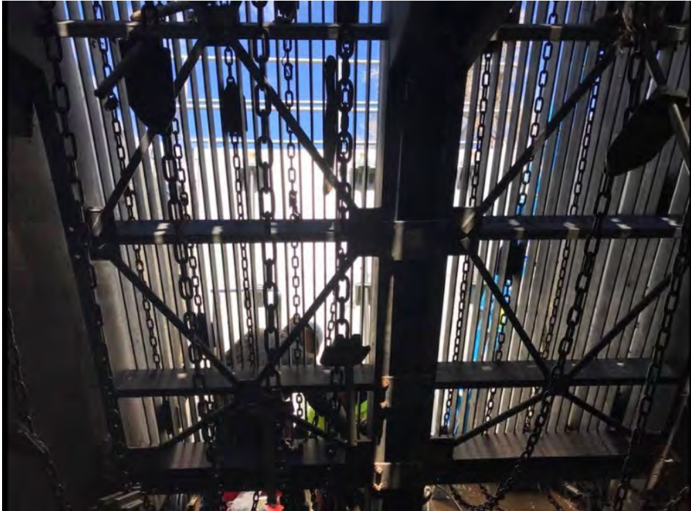
Glendale Treatment Plant Inlet
