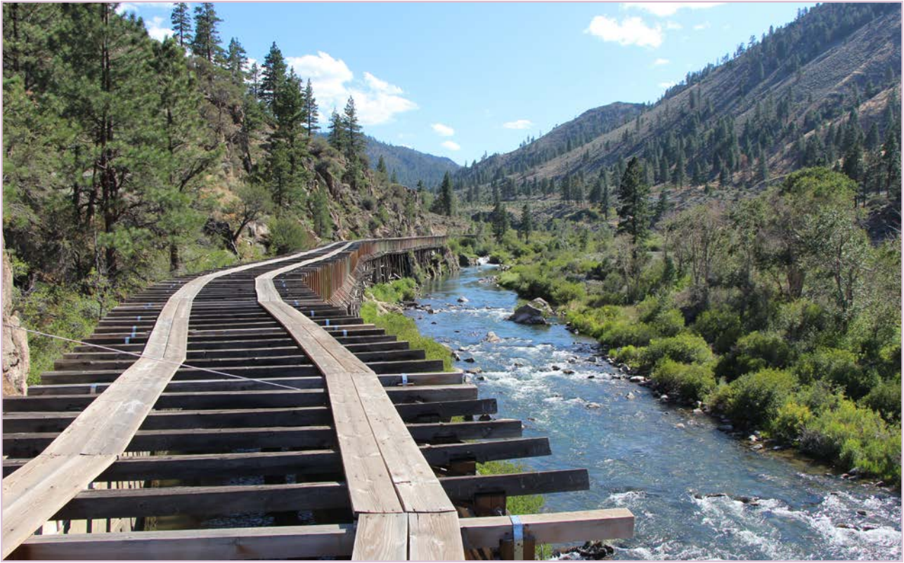
HYDROELECTRIC FLUME ALONG THE TRUCKEE RIVER
