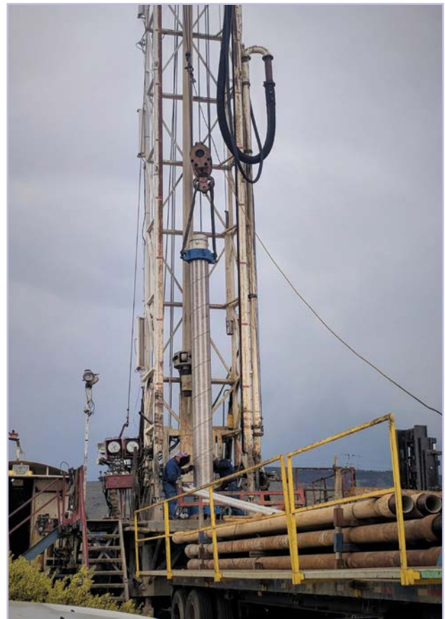
DRILLING A NEW PRODUCTION WELL
