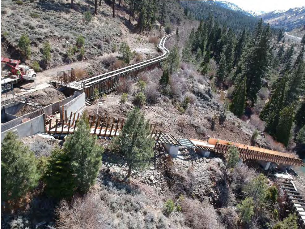
Fleish Spill Structure Reconstruction Project
