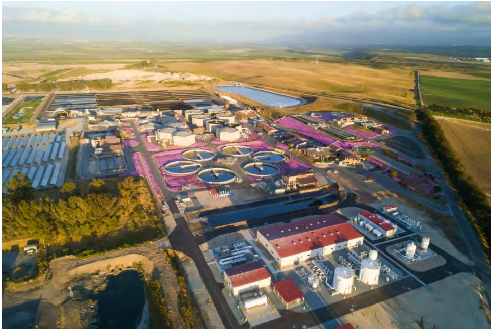
The Pure Water Monterey regional treatment plant. (Courtesy Monterey One Water)
