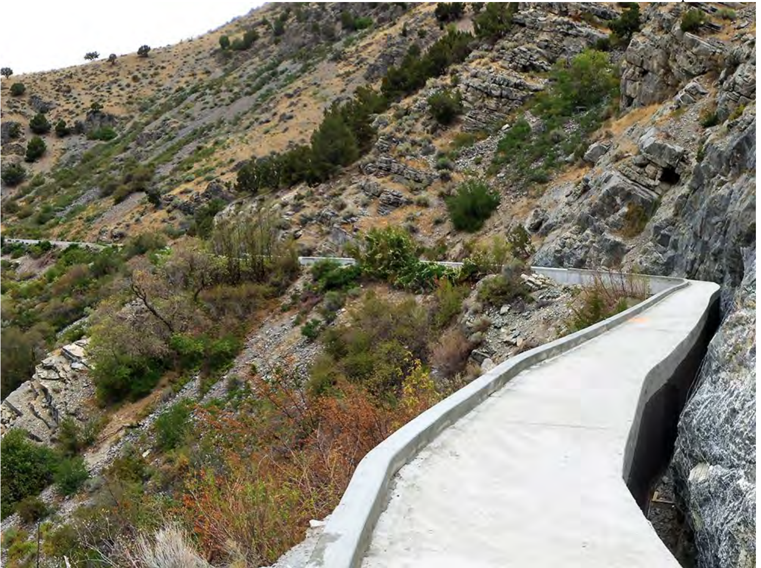
PHOTO/J-U-B ENGINEERS: This picture from the J-U-B website is from a project in Utah in which the firm enclosed six miles of open canal to restore irrigation water to shareholders lost from a breach. The company is also the contractor for the Steamboat grant.
