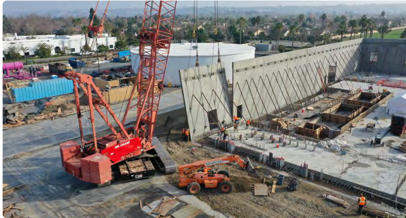
Foundation walls are lowered into place at the Pure Water Oceanside facility. Photo: Jeremy Kemp/City of Oceanside
