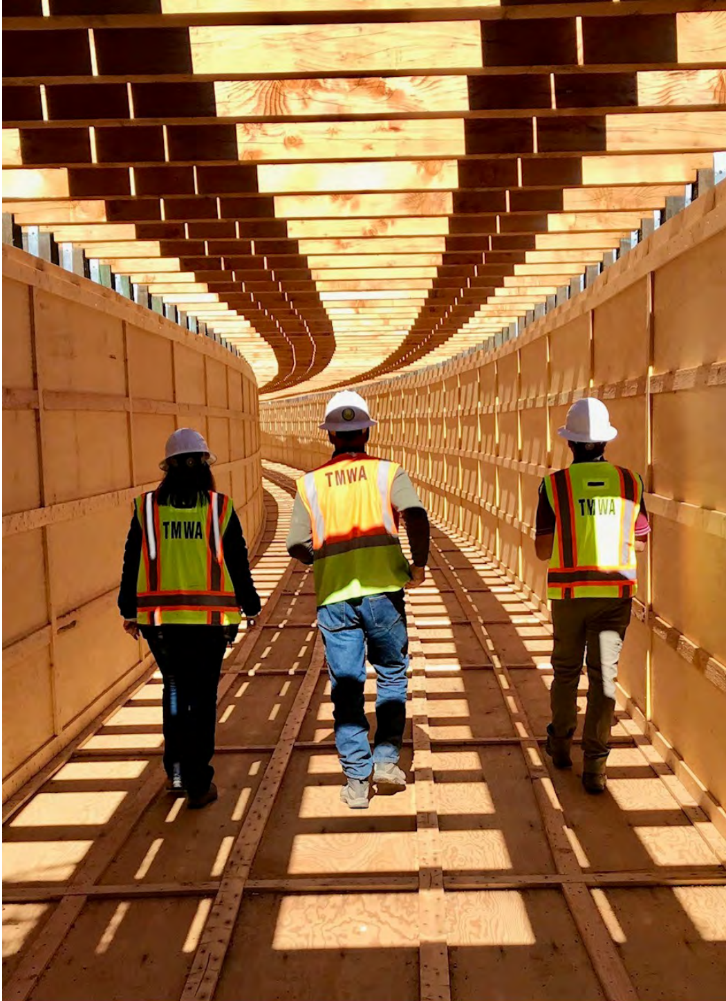
Photo: Washoe Flume Reconstruction
