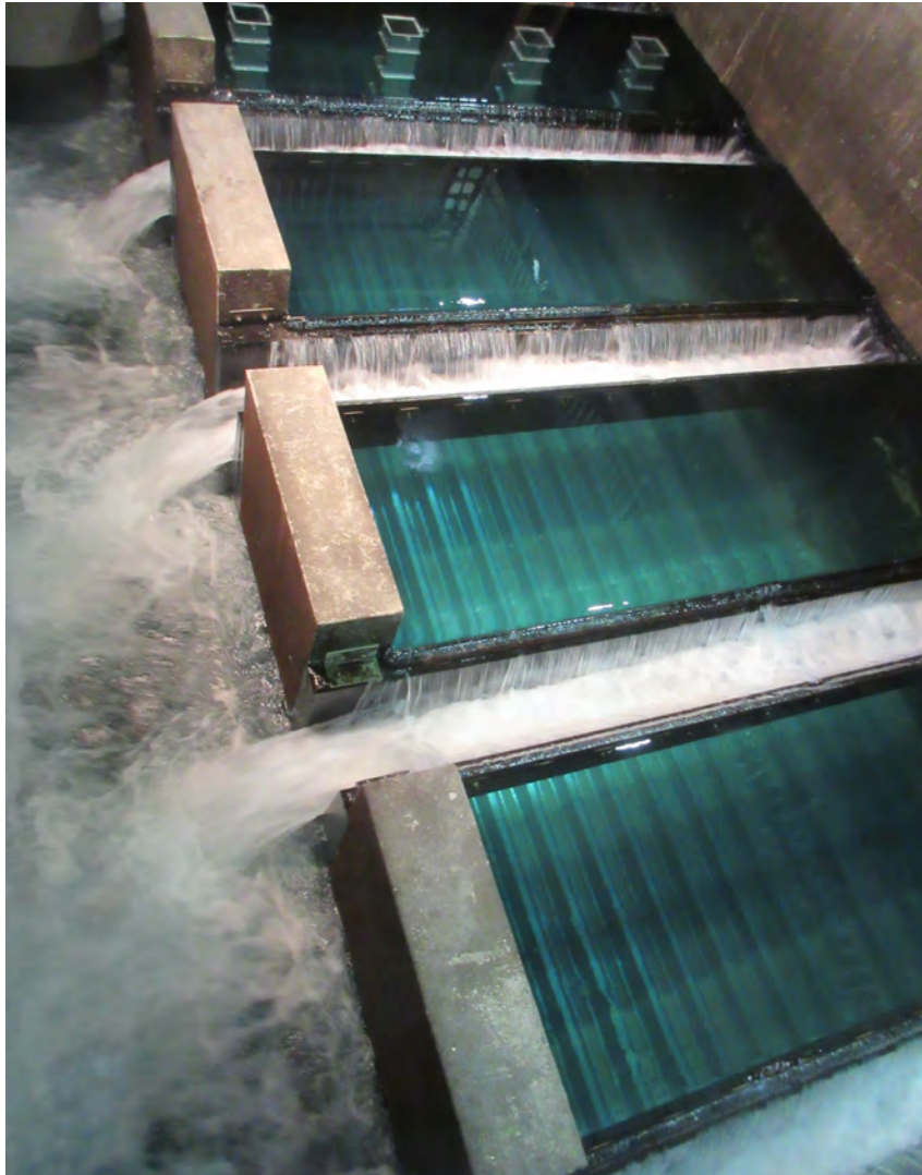
Photo: Chalk Bluff Filter Underdrain System
