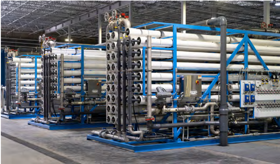
This facility in Oceanside, California turns recycled water into potable water by running it through filtration tubes.
