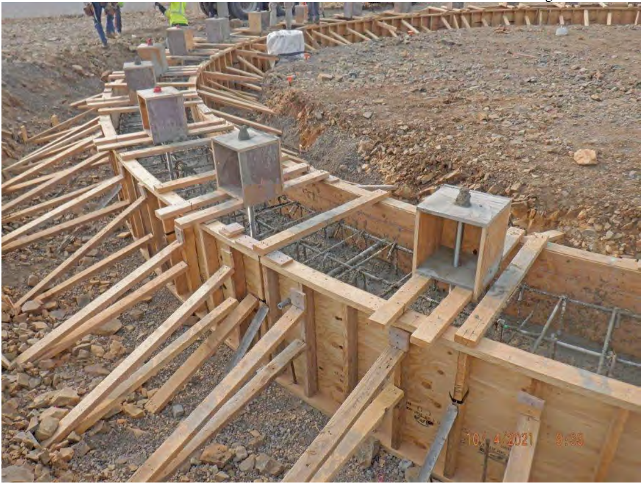
Concrete forms mark the start of construction of a half-million-gallon steel tank at the highest point along the pipeline, about 3.5 miles east of Sparks, Nev. Image by Troy Rasmussen, courtesy of Farr West Engineering
