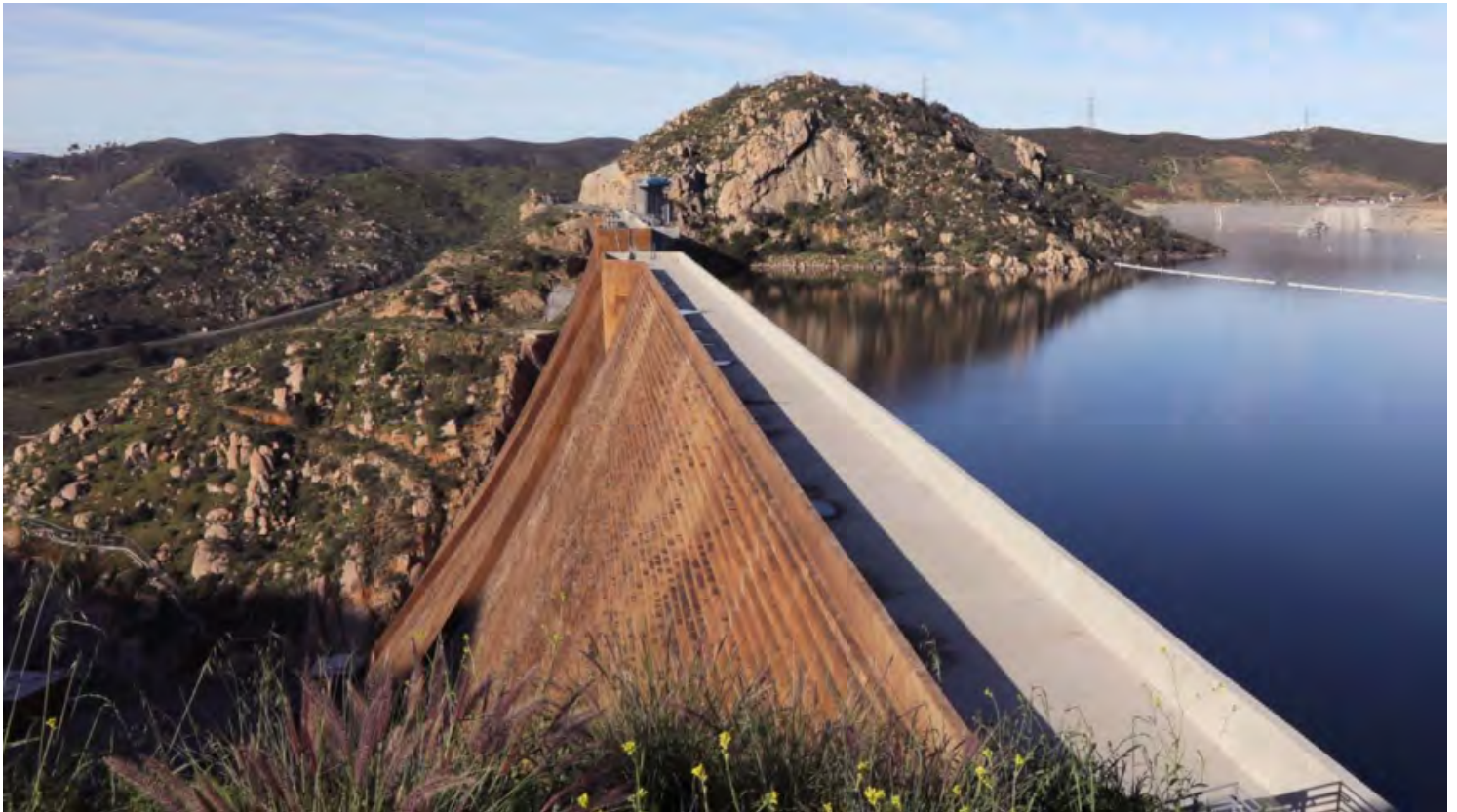
The San Vicente Dam in East County San Diego, north of Lakeside. The San Diego County Water Authority raised the dam 117 feet in the early 2010s, giving the region better water storage capacity. (Photo: SDCWA)
