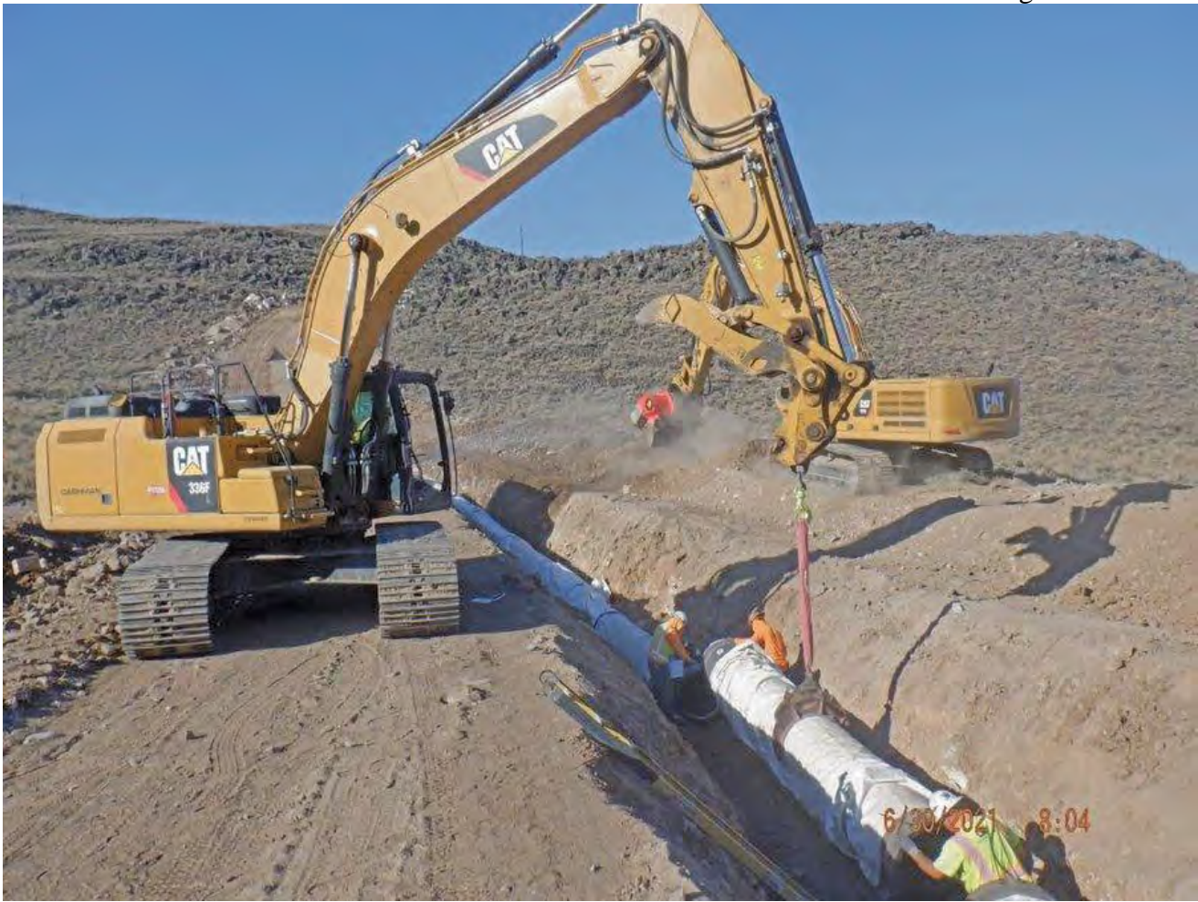
Q&D Construction installs a 24-in.-dia ductile iron pipeline that will move 4,000 acre-ft of water per year 16 miles to the Tahoe-Reno Industrial Center, where it will help cool servers at Switch data centers, among other uses.
