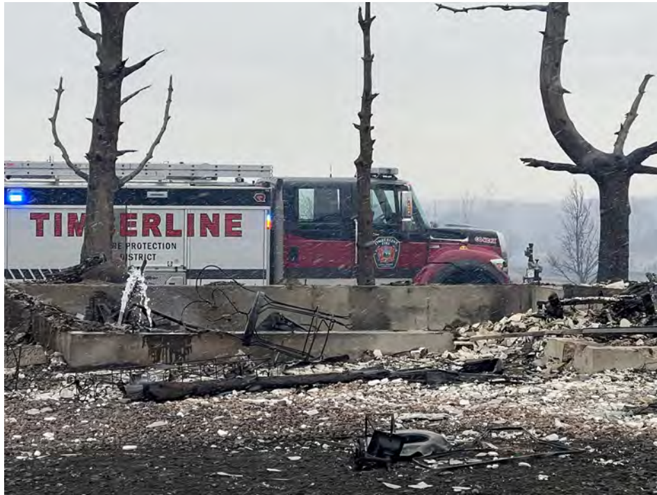
The entire Sagamore neighborhood in Superior, Colorado, was destroyed during the Marshall Fire in late December 2021. This photo shows water discharging from an open pipe into the foundation of a burned property. (Courtesy of Brad P. Wham)
