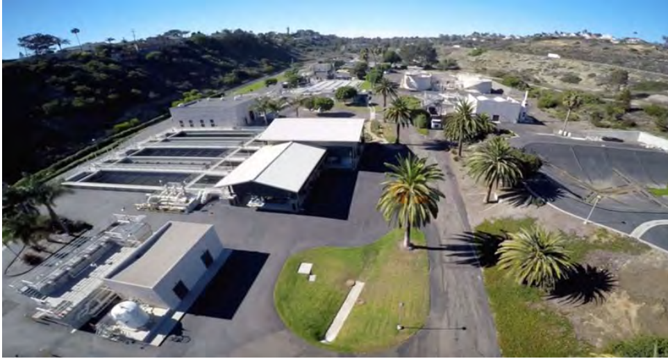
Recent construction of advanced water treatment facilities at the San Elijo Water Reclamation Facility allows for increased recycled water production. Photo: Courtesy SEJPA
