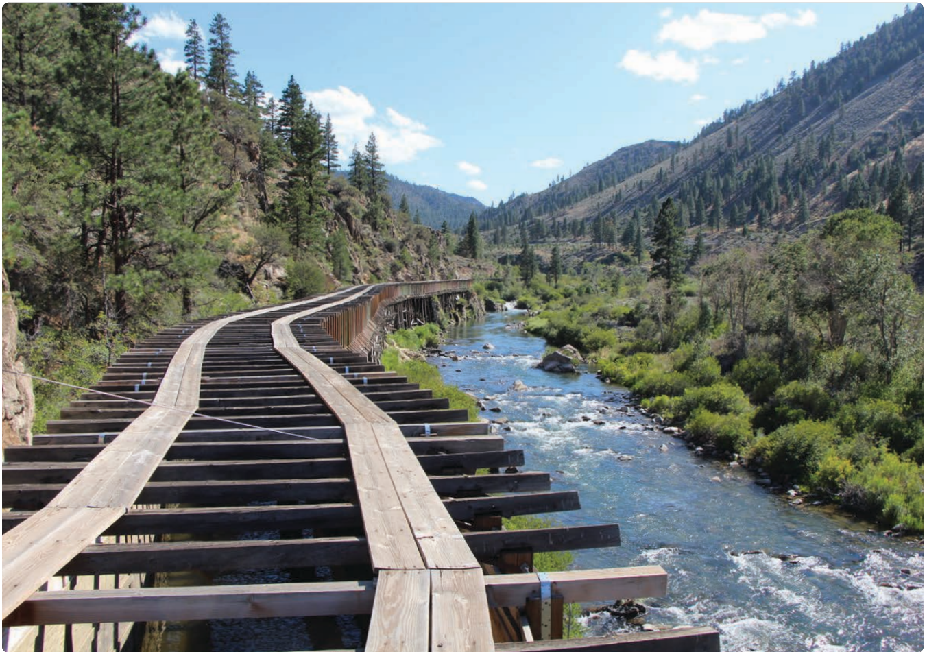
Fleish Hydroelectric Plant flume conveyance along the Truckee River.
