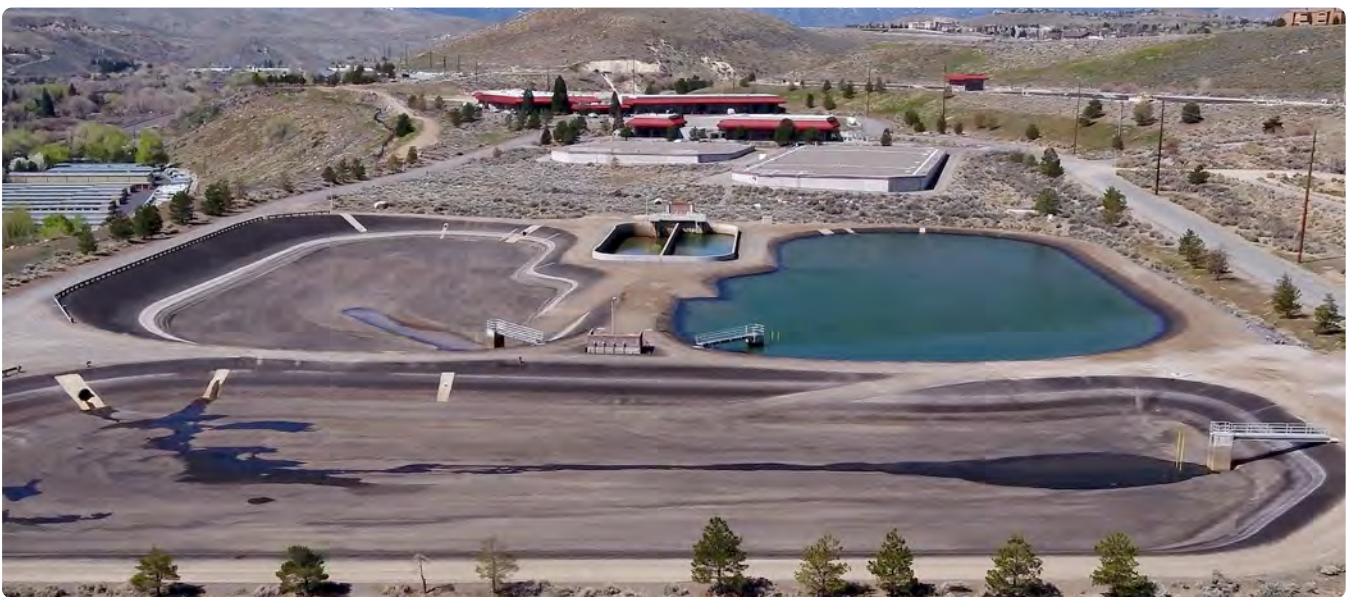
Chalk Bluff Water Treatment Plant
