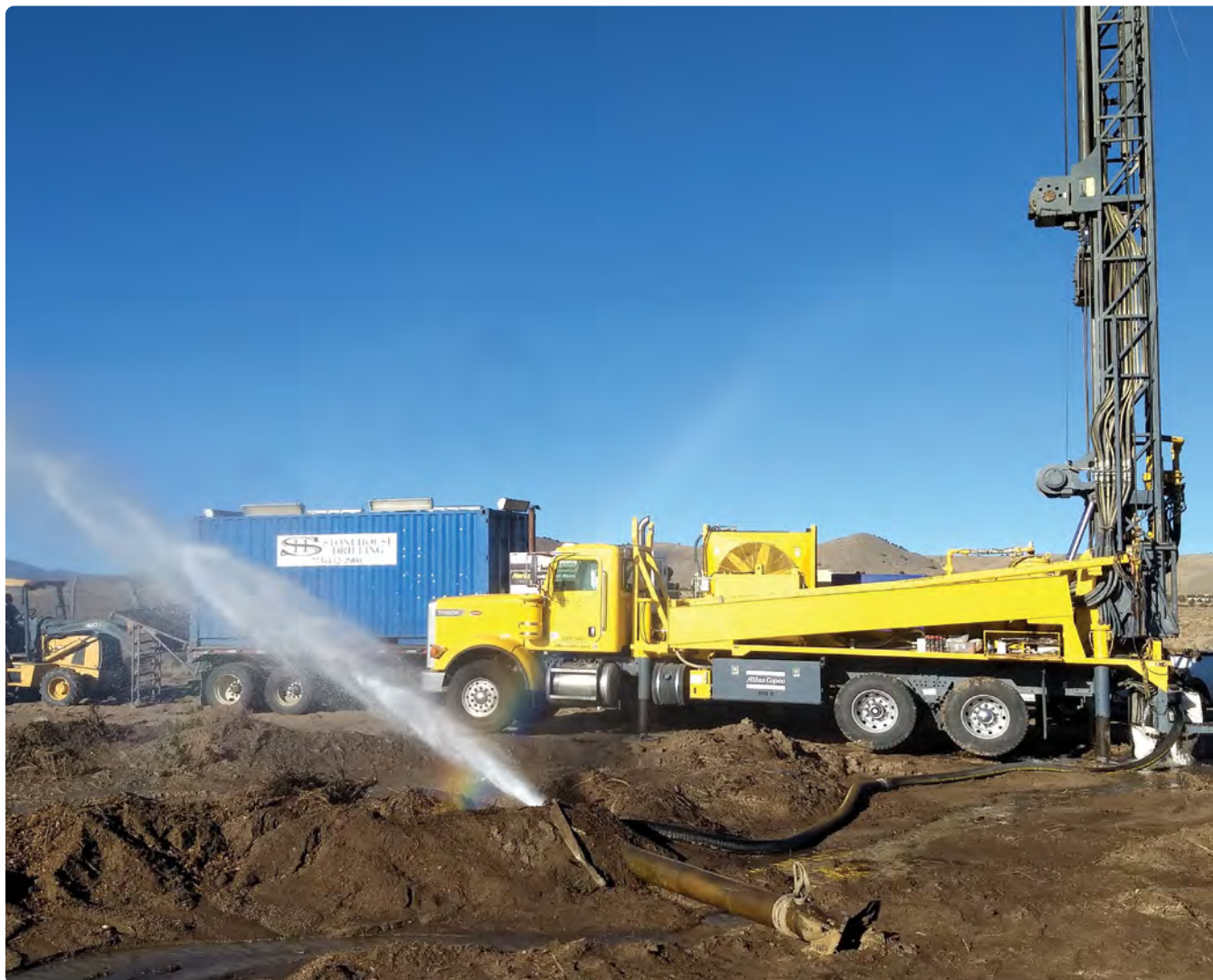
Drilling at American Flat
