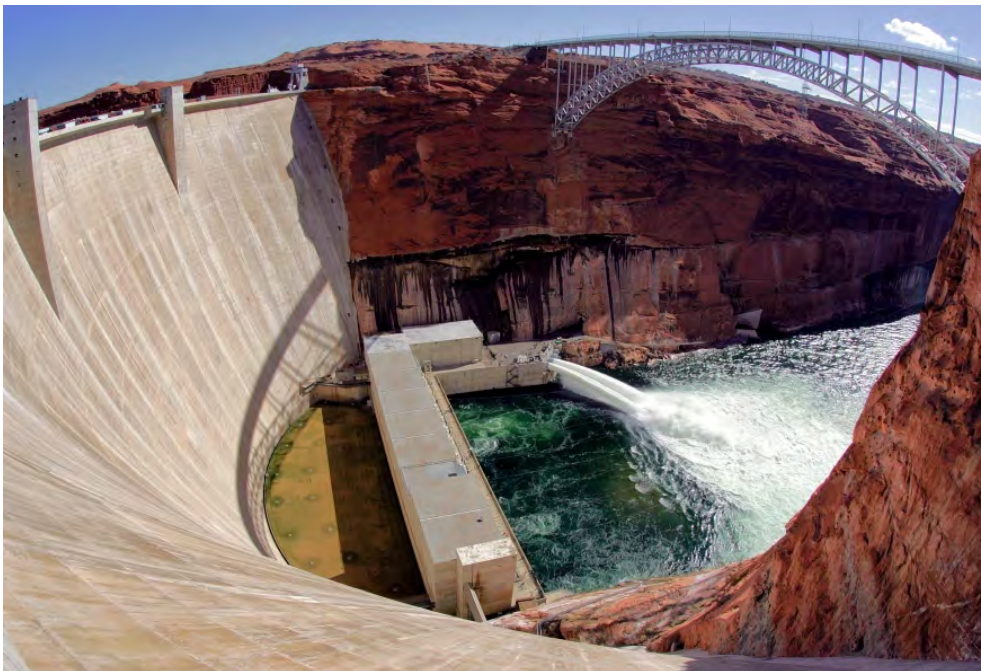
Water flows from the No. 1 and No. 2 jet tubes as seen from atop the Glen Canyon Dam, March 5, 2008, in Page, Ariz. (AP Photo/Matt York, File)
