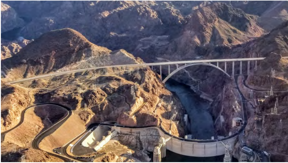
Hoover Dam, shown in an aerial view of the Nevada-Arizona state line. (Duncan Phenix / 8NewsNow)
