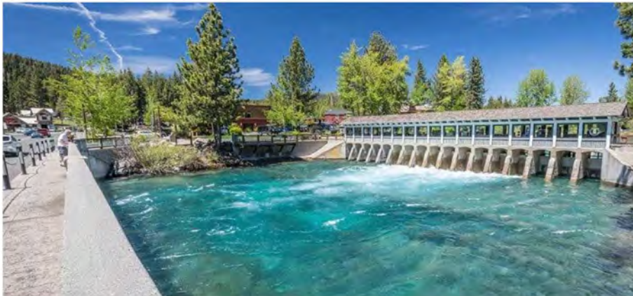
The dam in Tahoe City receiving a rapid influx of water from the ongoing storms. Photo taken from Fanny Bridge.
