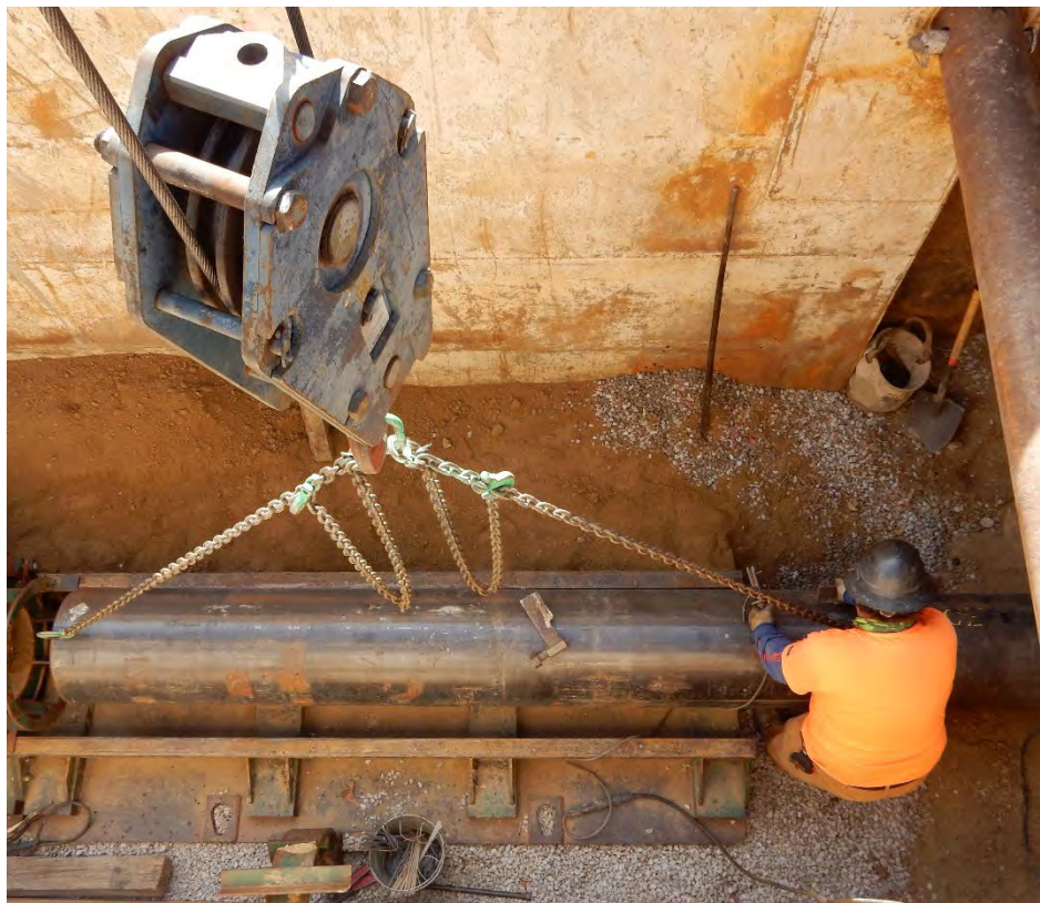
Bartlett Main Replacement
