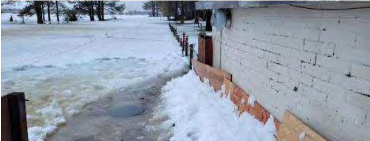
Bellevue pump station temporary containment
