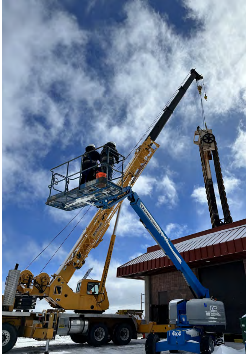
Photo: Traveling Screen 1 Rebuild, Chalk Bluff Water Treatment Plant
