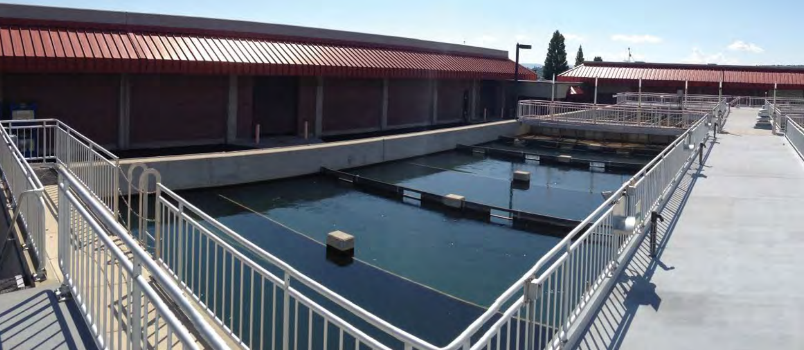
Chalk Bluff Water Treatment Plant
