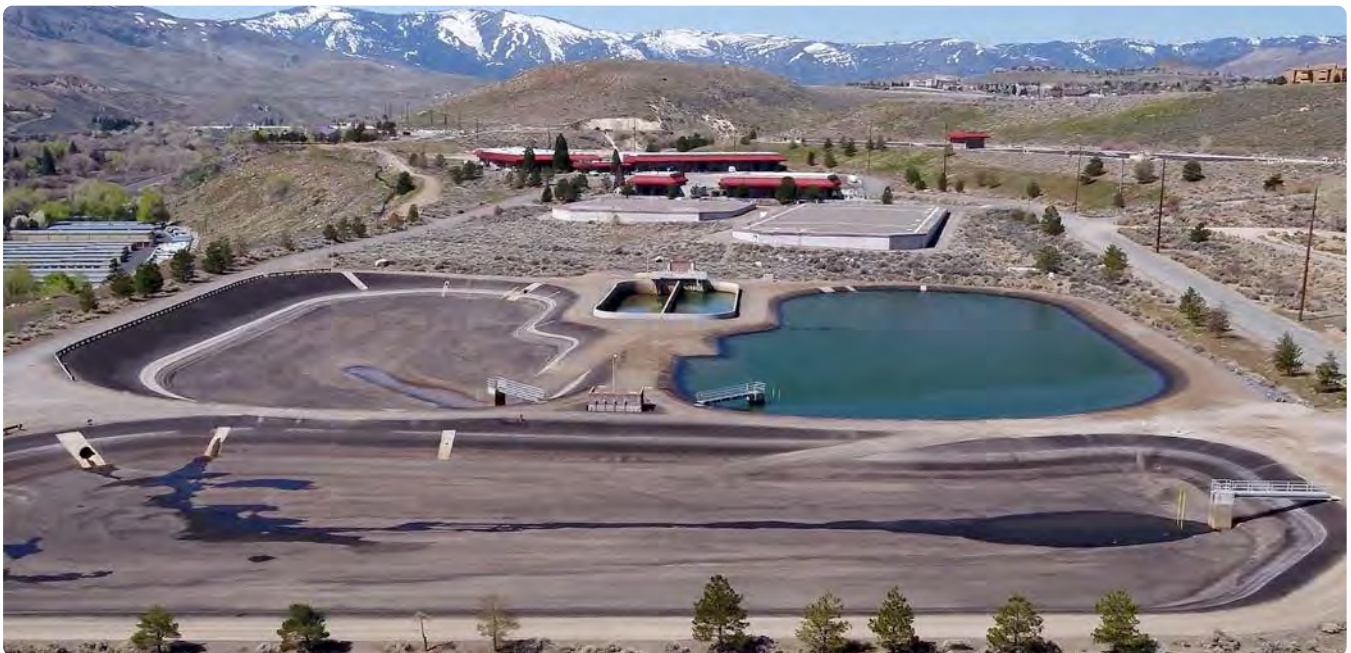
Chalk Bluff Water Treatment Plant
