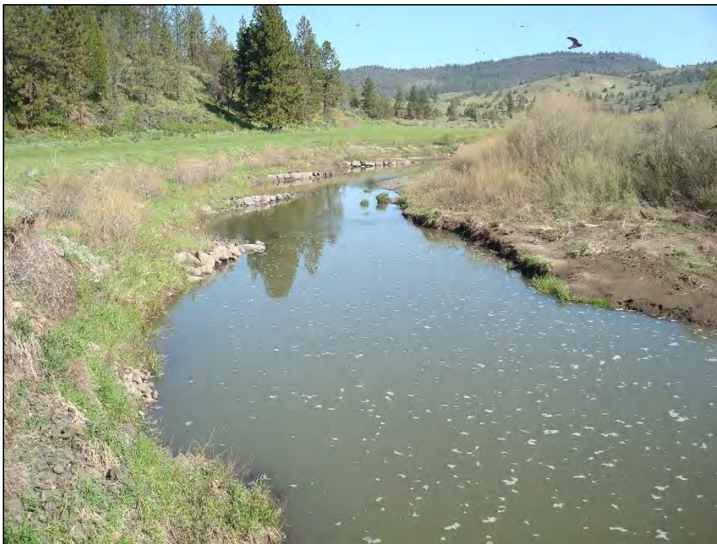
Series of j-hook vanes protecting RB along Pit River, Modoc County, CA
