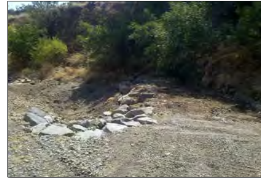
J-Hook Vane in dry stream showing scour pool below
