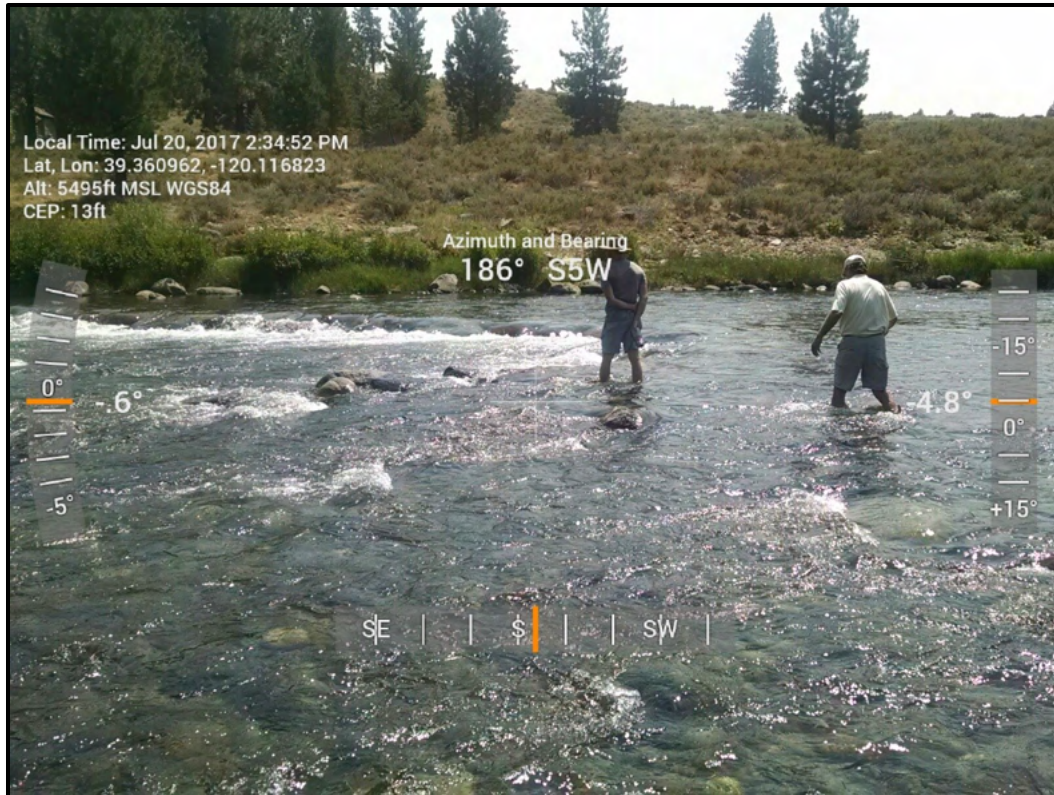
J-Hook Vane on Truckee near Glenshire Drive. ( Note convergent flow pattern.)
