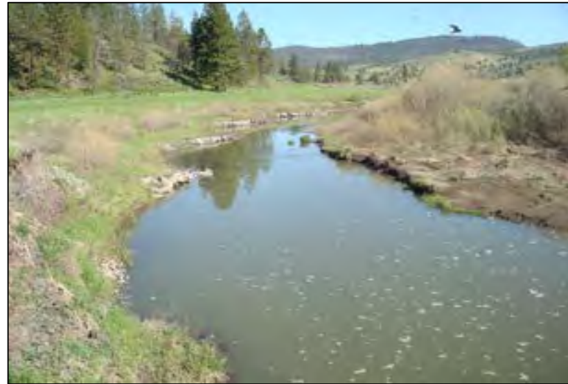
J-Hook vane series along Pit River meander - Modoc County, CA
