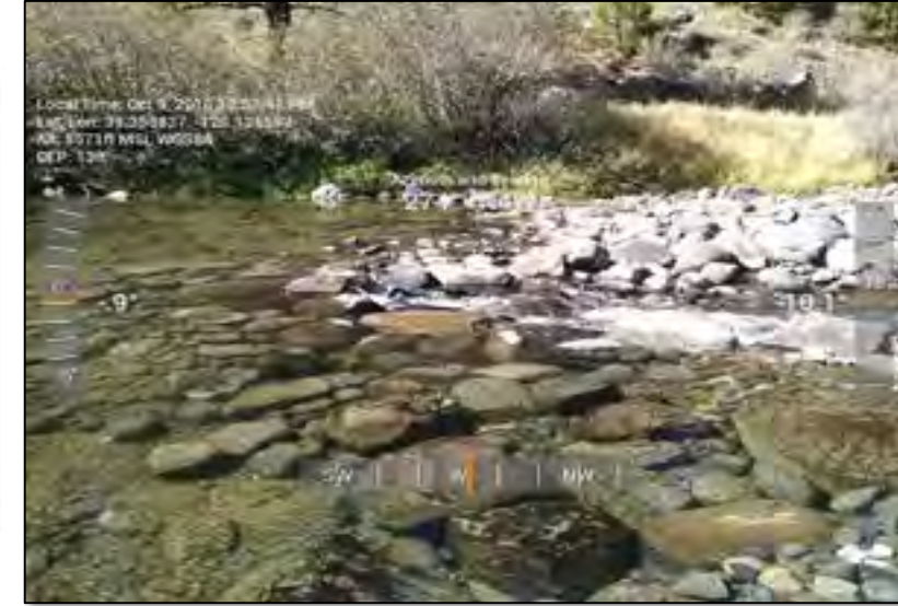
J-Hook Vane on Truckee River
