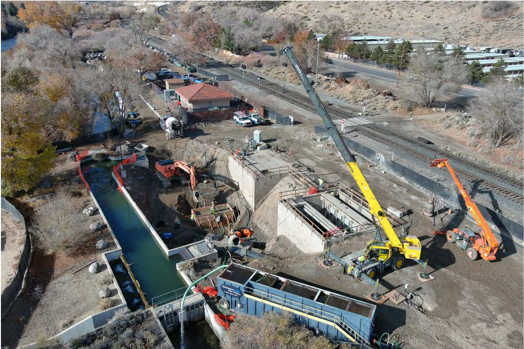
CURRENT STATE OF CONSTRUCTION NOVEMBER 2023
