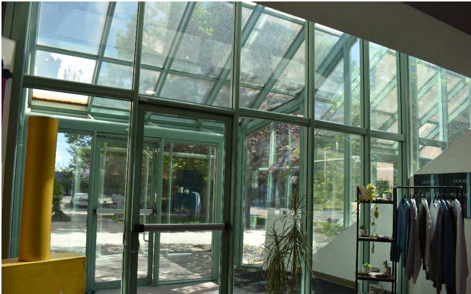
INTERIOR VIEW OF THE MAIN ENTRY IN THE SUBJECT BUILDING
