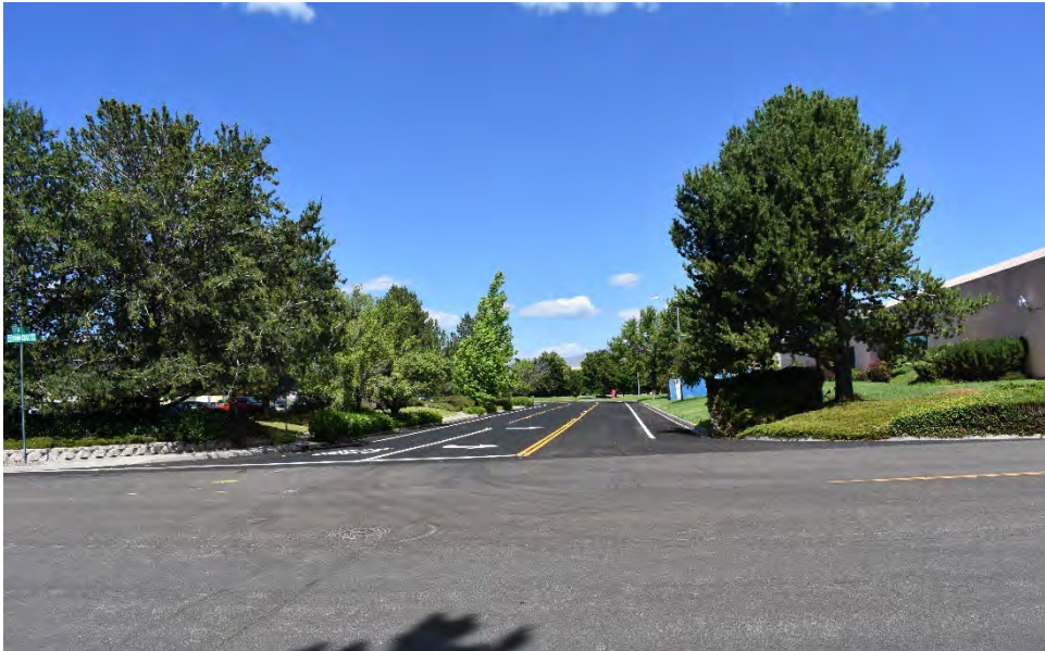
VIEW LOOKING WESTERLY TOWARD WALL STREET AT ITS INTERSECTION WITH FINANCIAL BLVD, WITH THE SUBJECT TO THE RIGHT
