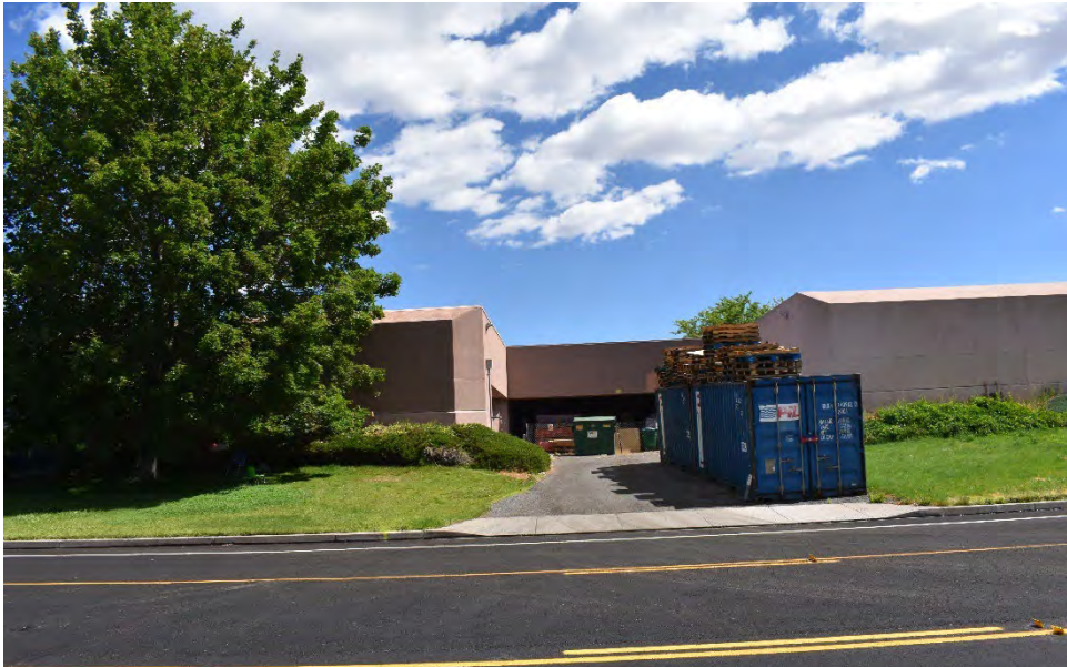
VIEW OF THE SUBJECT’S LOADING DOCK LOOKING NORTHERLY FROM WALL STREET
