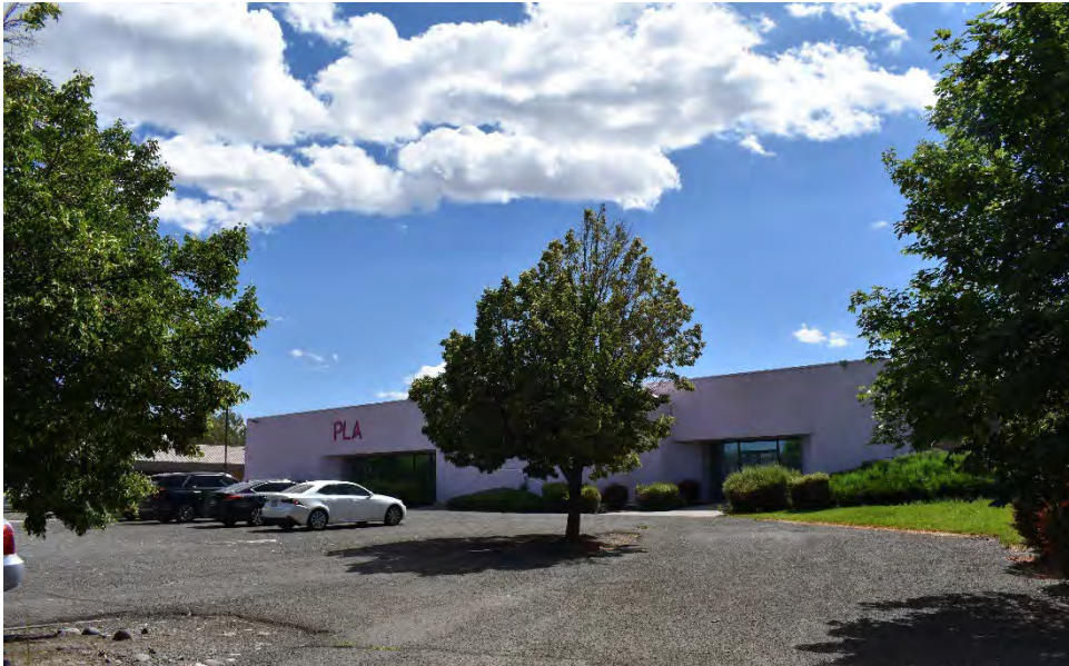
VIEW OF THE SUBJECT BUILDING FROM THE WEST (REAR) PARKING AREA
