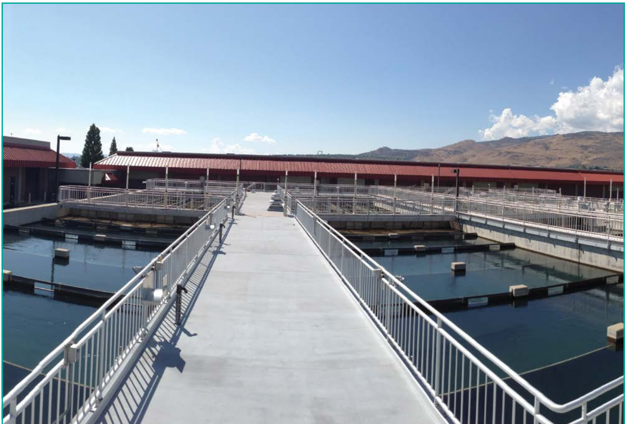
CHALK BLUFF WATER TREATMENT PLANT
