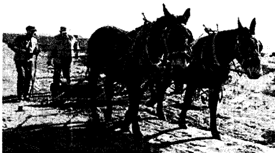
Zoom CID board members tried their hand at using this historic Fresno scraper, which was powered by a mule-team at the irrigation district's groundbreaking ceremony for the canal conduit rehabilitation project. / Photo by Richard Booth
